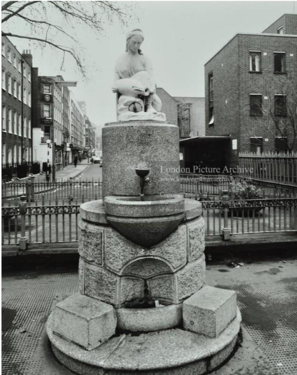
*Fig 03 – Photograph of the Guilford Place Drinking Fountain in 1971. Note that the original floral tap had been replaced with a cup-type fountain. Note also the relative lack of damage to the granite base at this time, and the ‘withered’ appearance of the marble jug’s handle.*
