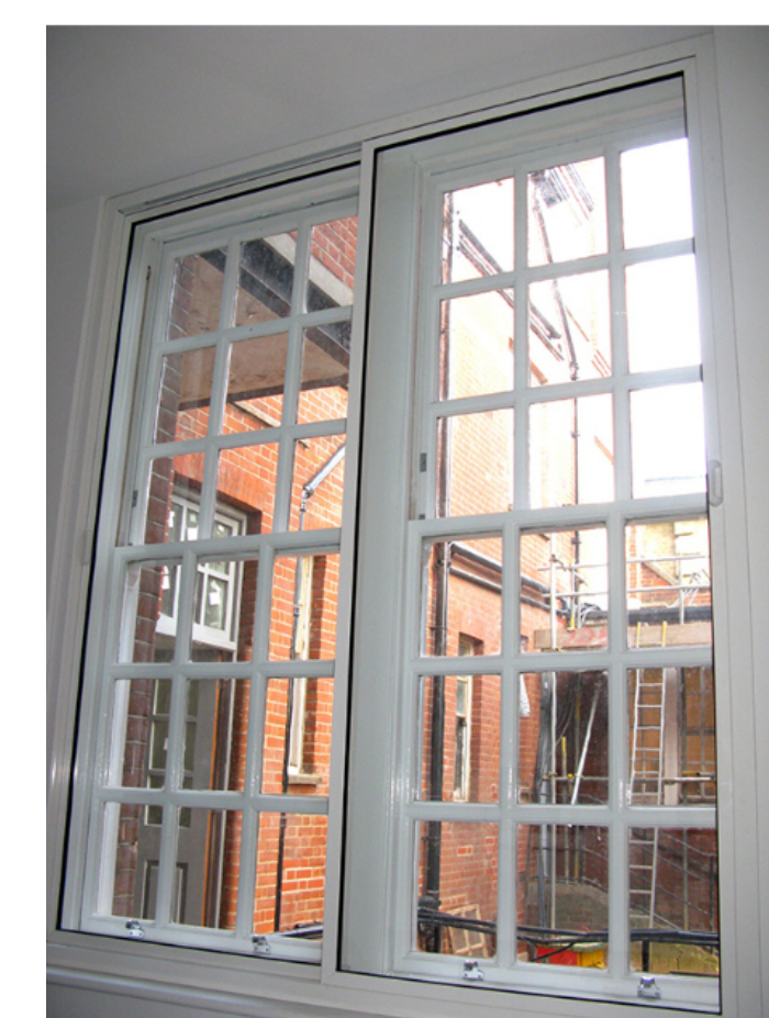
Selectagaze secondary glazing - Typical Installation
