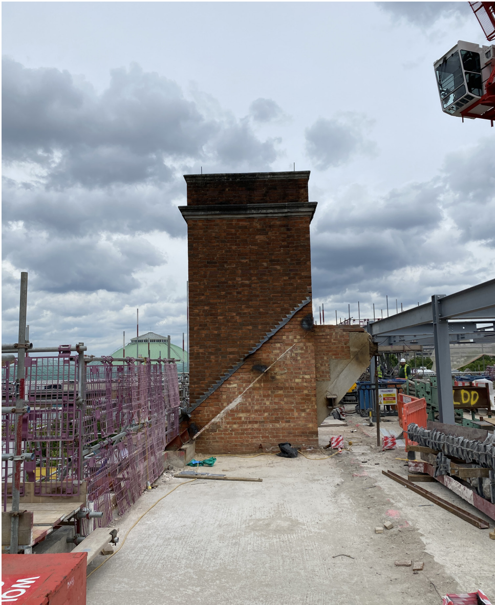
Existing Site Image
