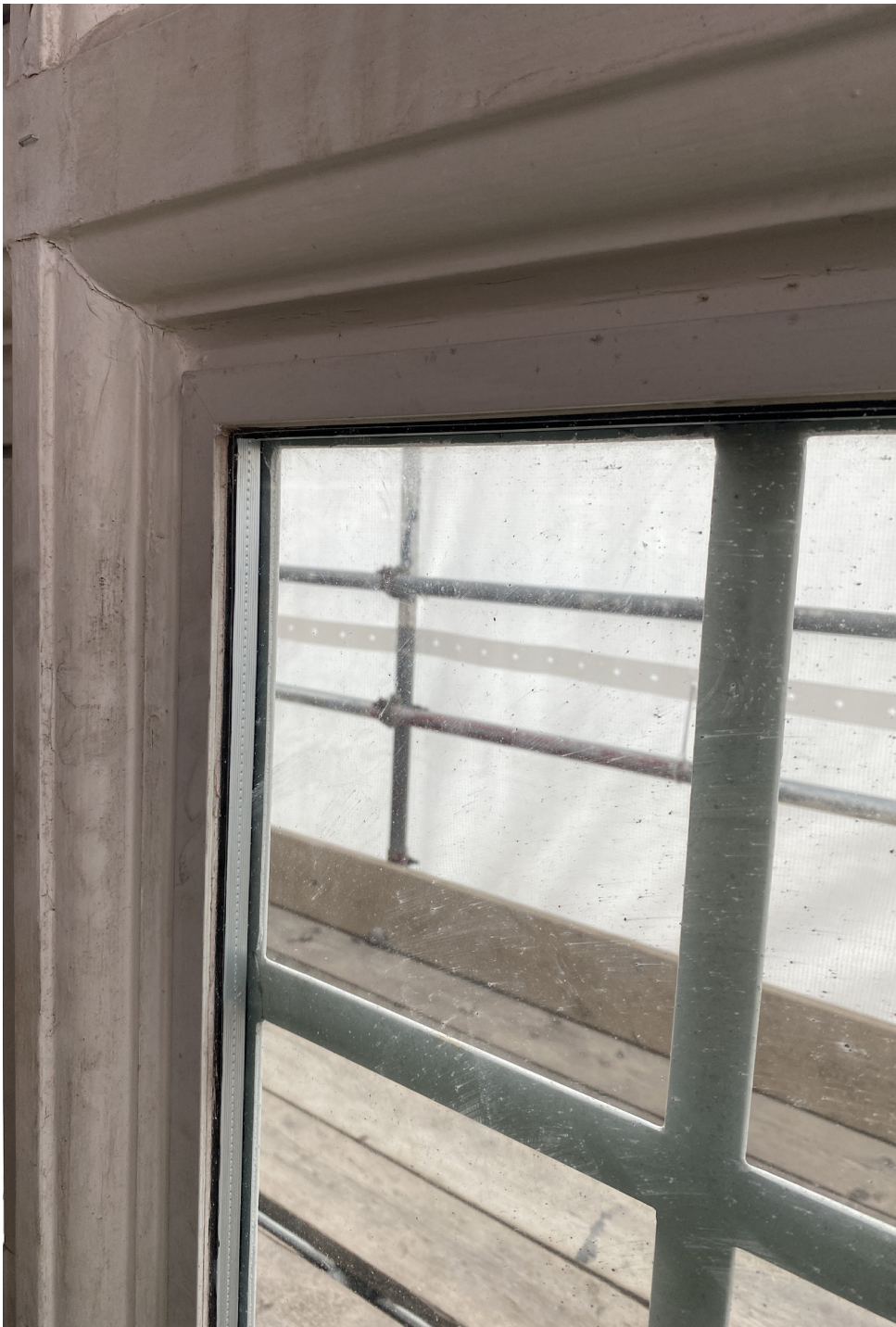
Existing Site Image
