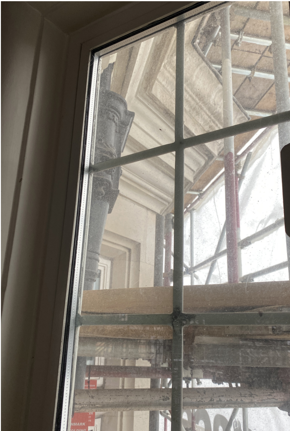
Existing Site Image
