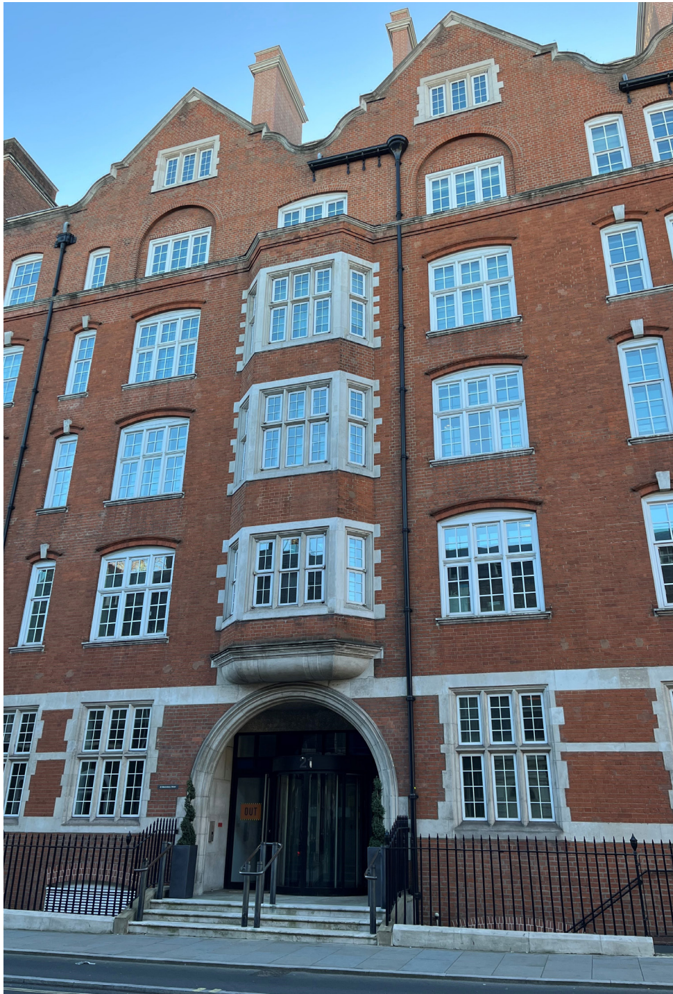
Existing Site Image
