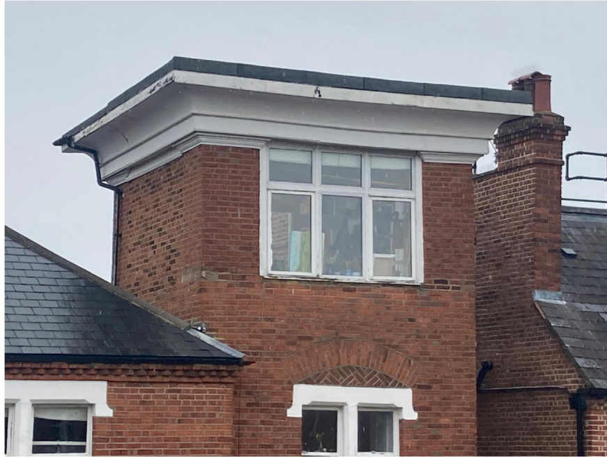
Above: The turret at No 56 today. It has been considerably altered over time with variations in bricks used on the street façade and flanks. The detailing of the capping cornicing either side of the window appear 19 th century but the main capping cornice has somewhat different detailing that might be later – as might that at No 58. However, drainage plans indicate that both towers were in place before 1929.
