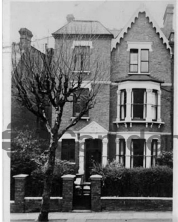
Above: Archival image of 49 Parliament Hill showing a pyramid slate roof with corbelled brick cornice at its eaves on the side wing. It is possible but no means certain that Nos 56 and 58 originally had similar roofs to their side wings with their 'towers' added in the early 20 th century.
