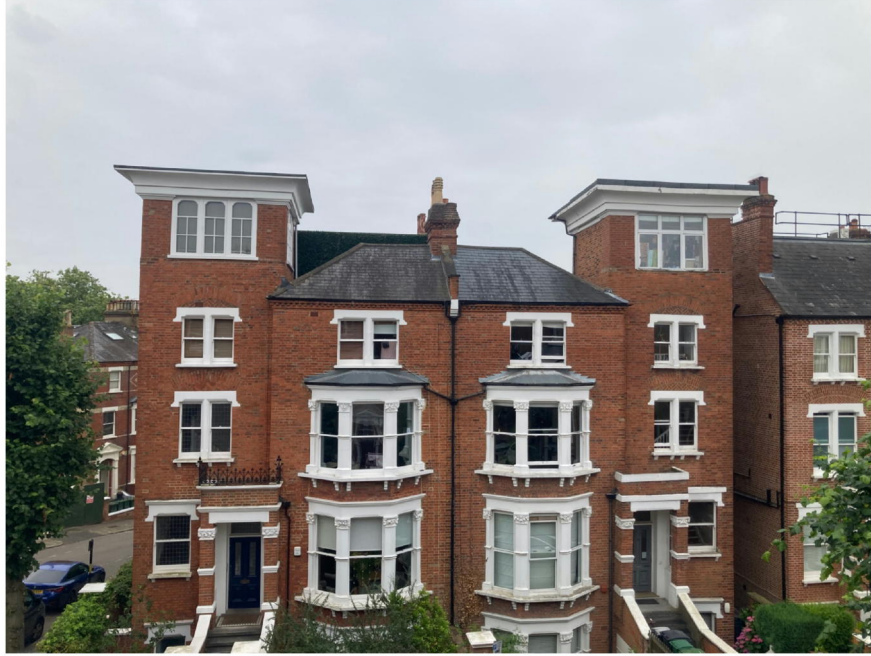
Above: Nos 56 and 58 are unique in the conservation area in having square corner turrets. They mix Italianate features such as these towers and the square porches with Gothic Revival elements such as mouldings and the corbelled brick cornices at eaves level.
