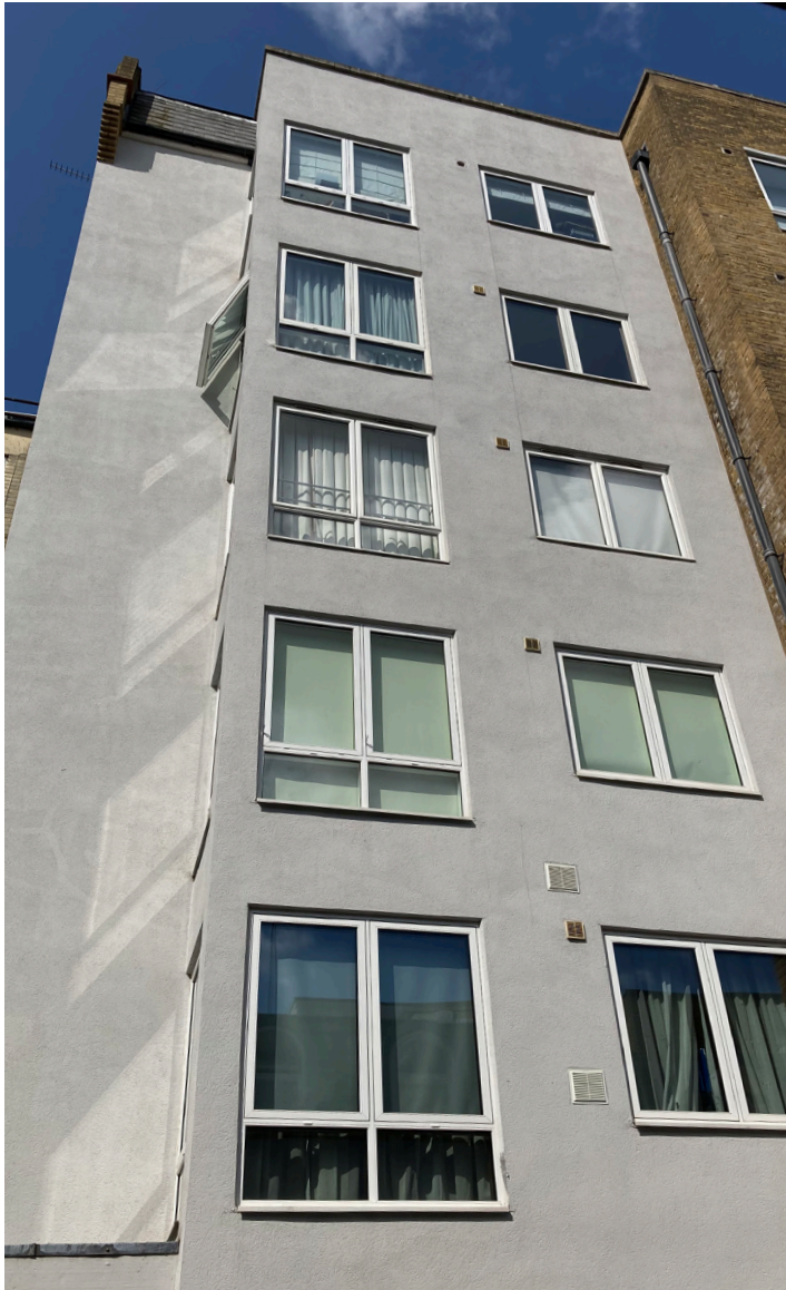
3a. East elevation - Existing external wall insulation
