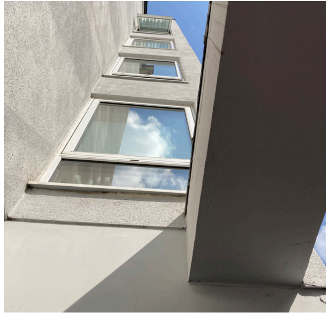
3b. Existing EWI on east elevation return
