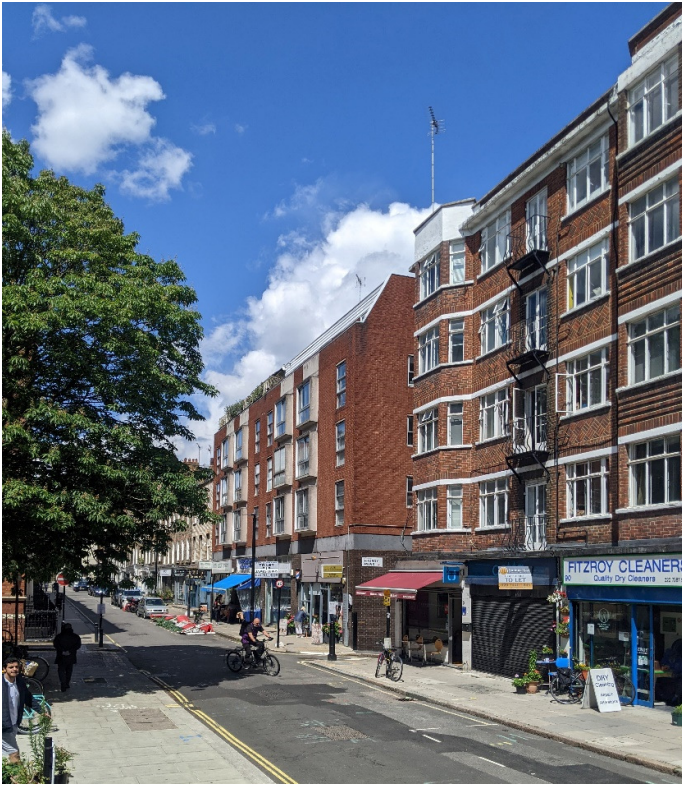
Existing – view north up Cleveland Street
