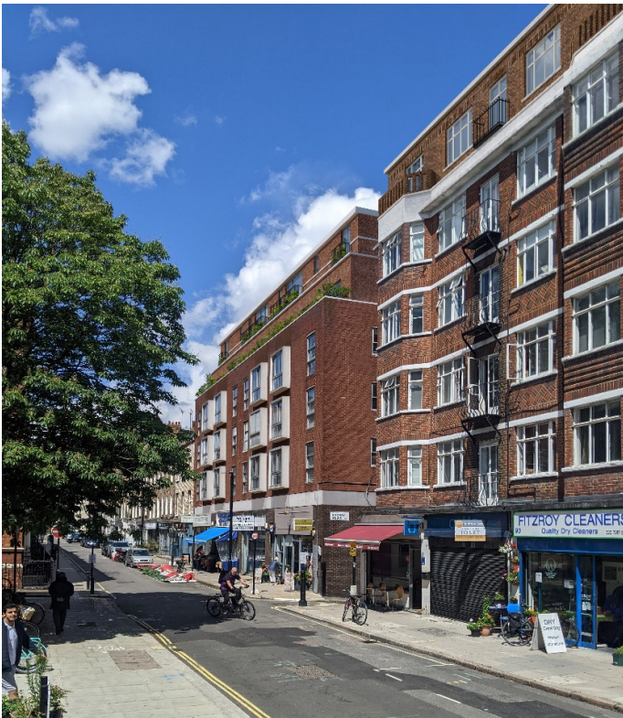
Proposed – view north up Cleveland Street (including new 5 th floor to Cleveland Court)
