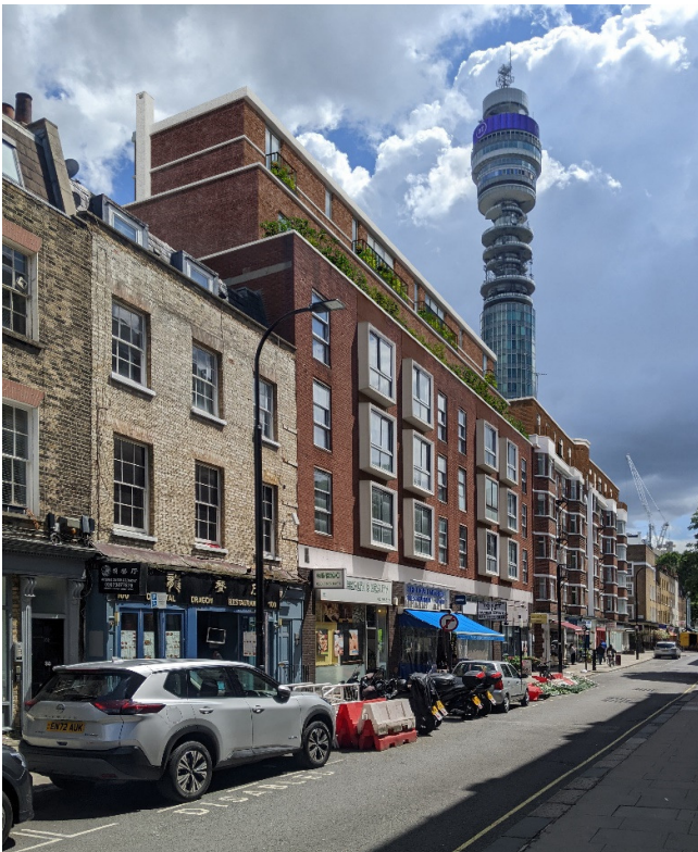
Proposed – view South down Cleveland Street (including new 5 th floor to Cleveland Court)
