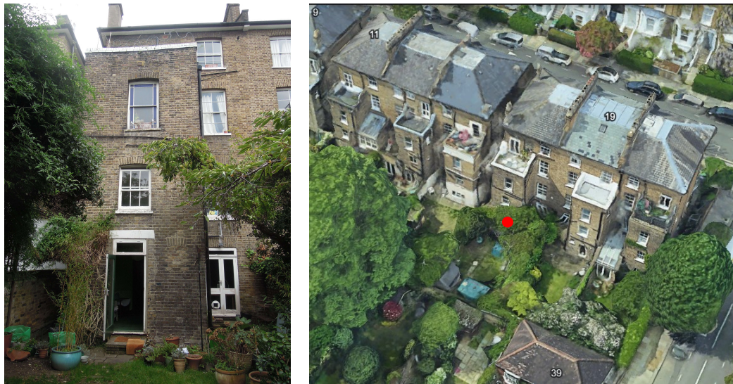
Fig 2: Existing rear south elevation and aerial view
