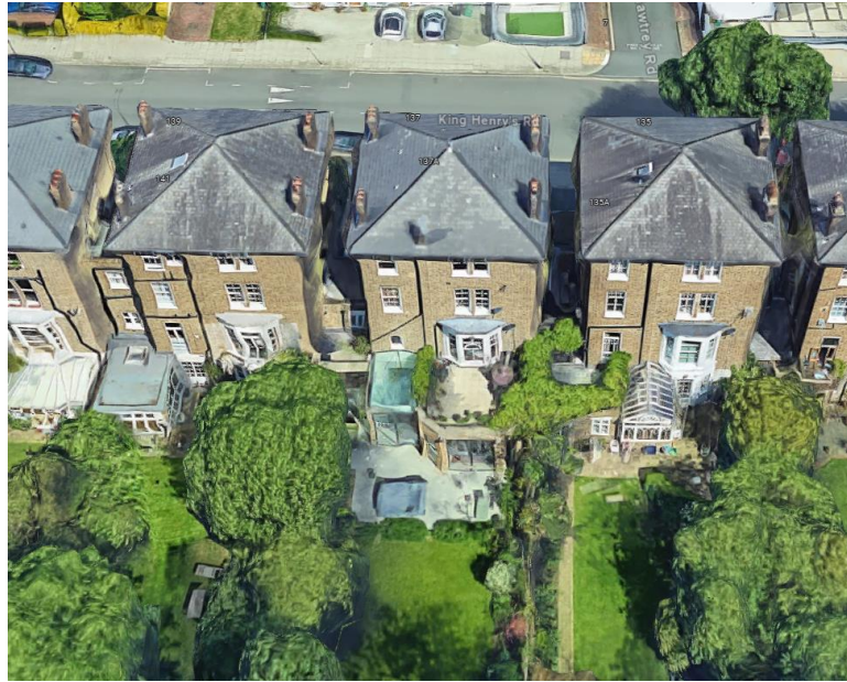
Figure 1. The rear of 137a King Henry's Road with a terrace in the middle from Google Aerial view
