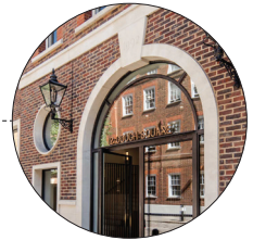
Bronze coloured, metal-framed windows
