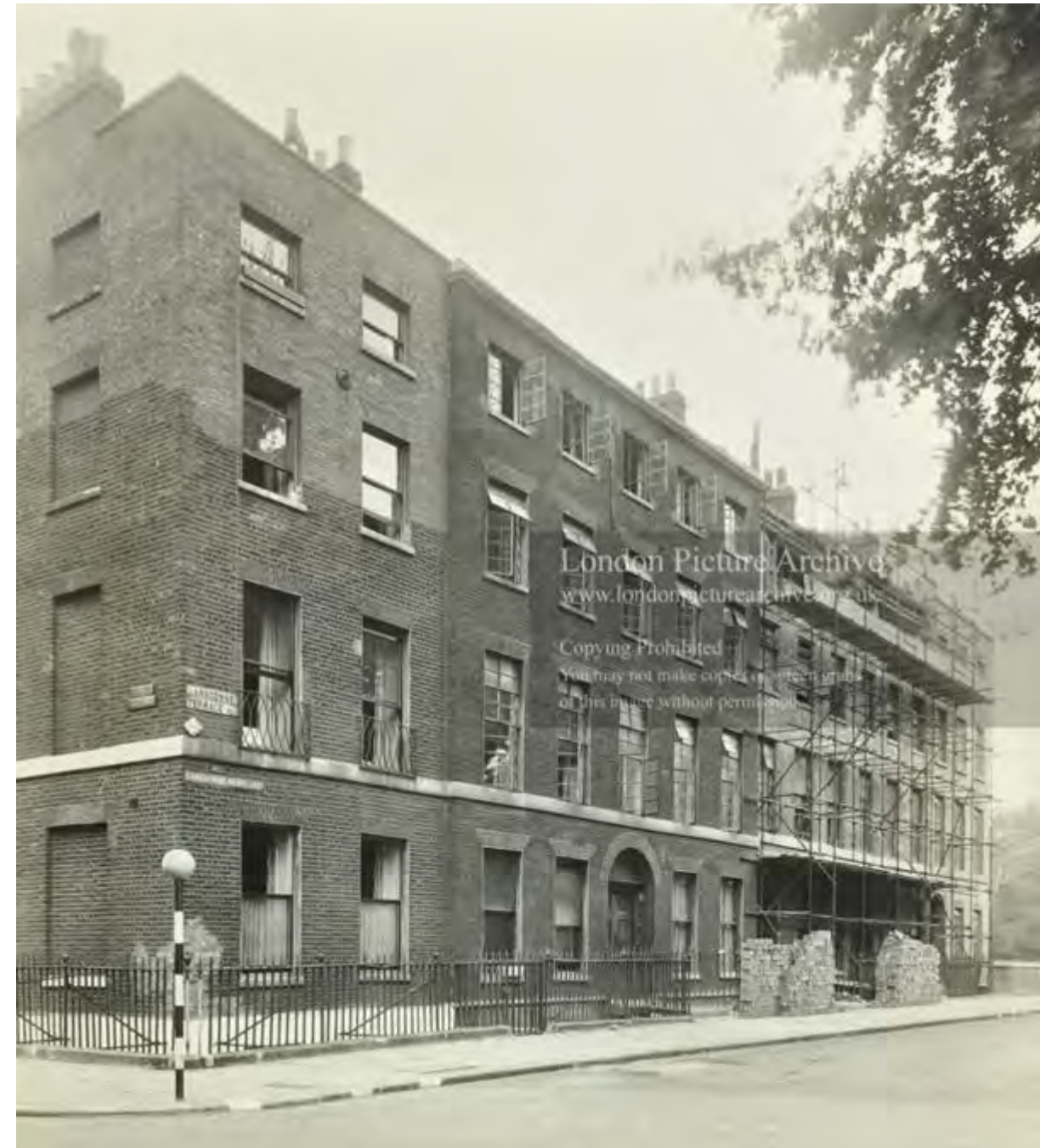
Figure 2 - 1940's photograph of Lansdowne Terrace showing rebuilding in progress.
