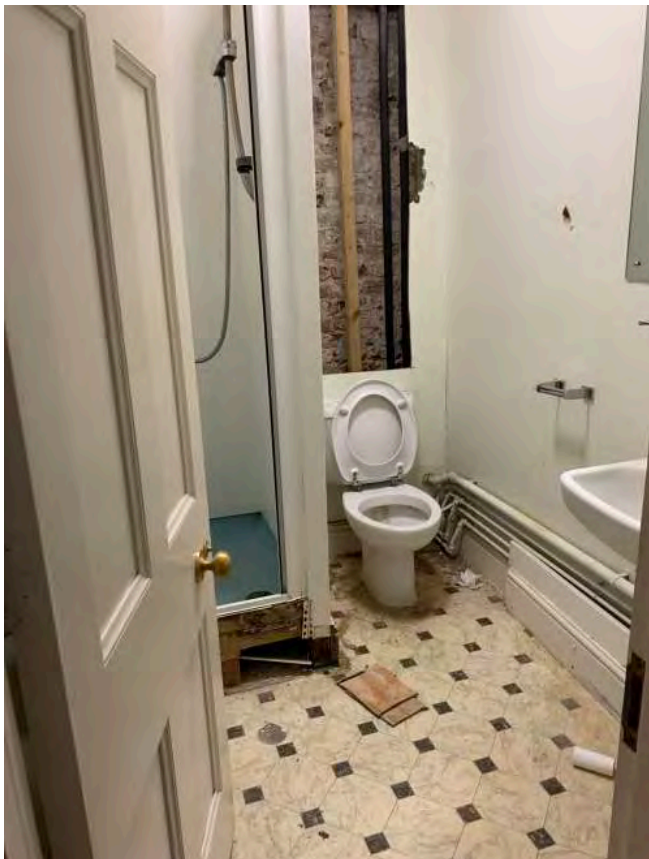
Bathrooms are cramped, in disrepair and many fixtures and fittings are at end of life
