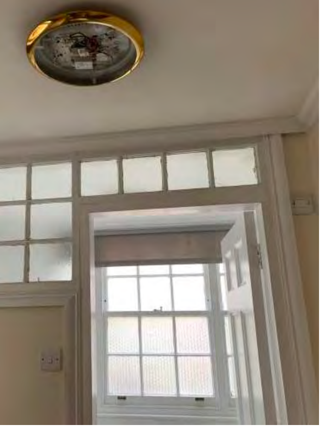
Internal windows required where outrigger layout blocks natural light to inner rooms
