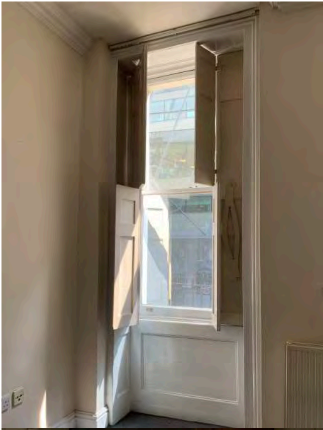
Original box shutters remain in Ground Floor primary room
