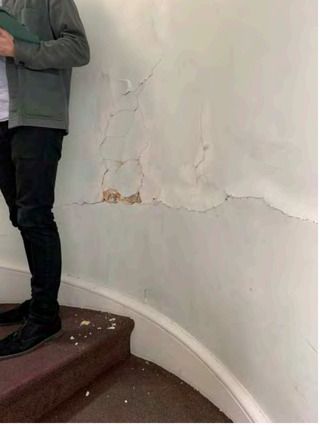
Damage to existing curved stair wall
