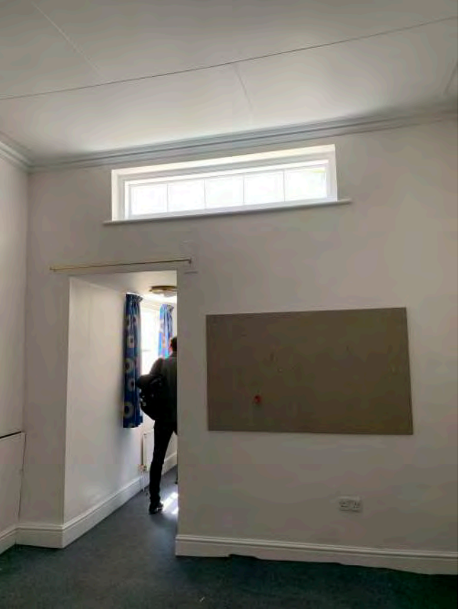
Outrigger layout causes inner rooms with limited natural light
