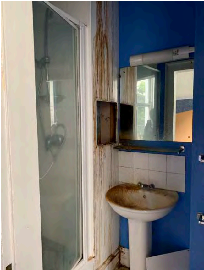
Bathroom blocks the original front door and is in sever state of disrepair
