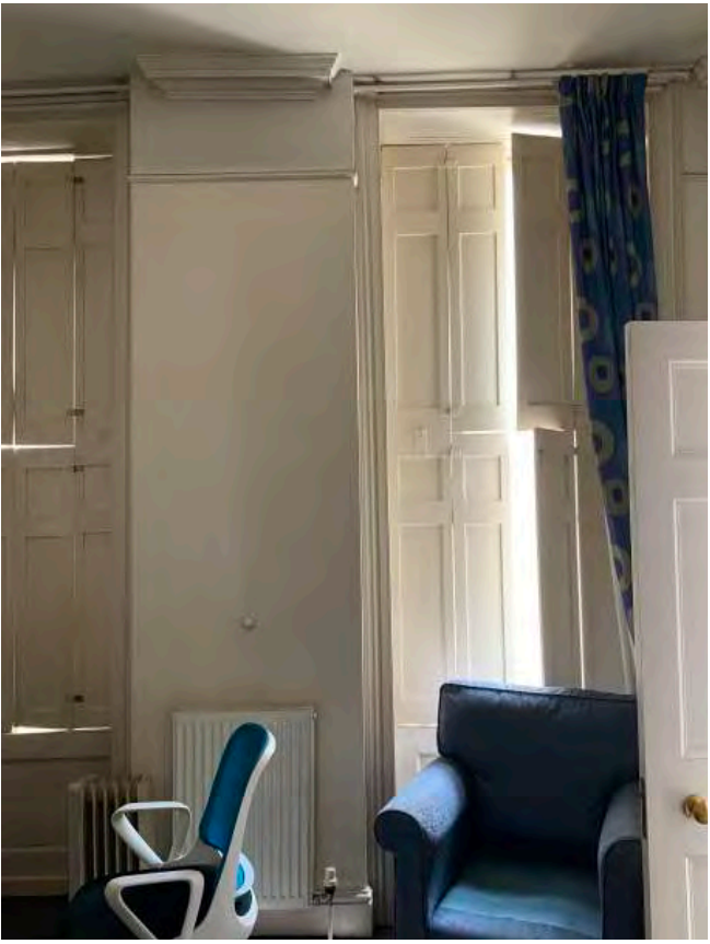
Original box shutters remain in 1st Floor primary room
