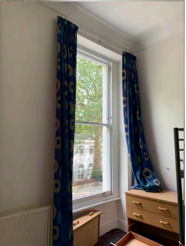
Modern single glazed sashes in historic openings. No surviving box shutters in Lansdowne Terrace.
