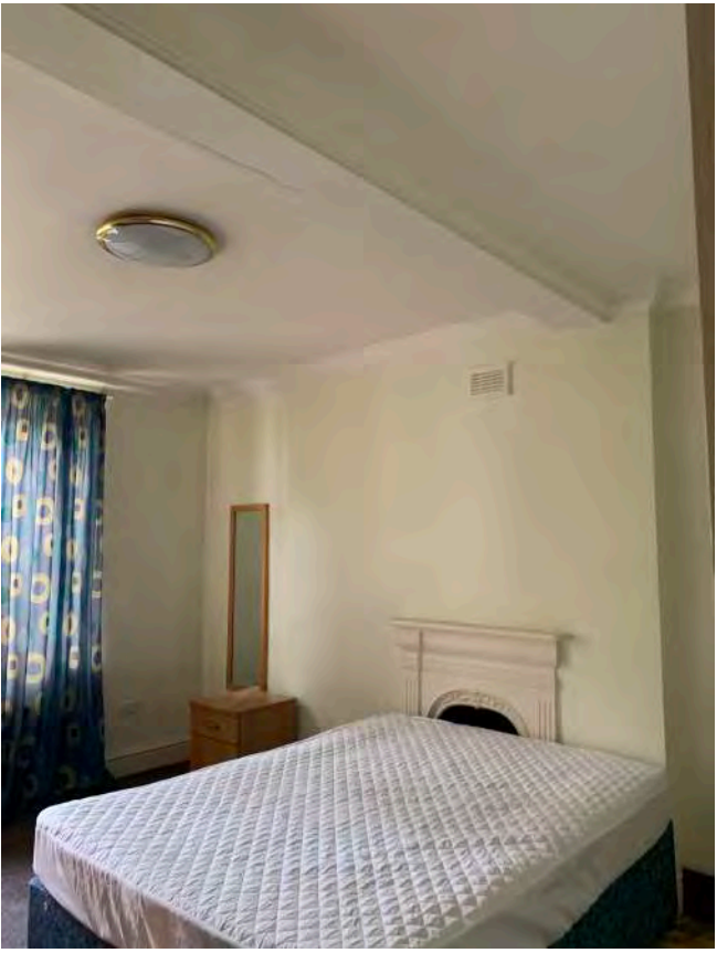
Downstand beams in second floor rear rooms indicate possible original structural layout
