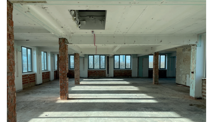
Structural beams to underside of slab, typical floor
