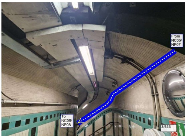
Figures 10 & 11: Proposed new cabling in the stairways and passages of the station. Proposed new CMS shown in blue. The CMS will be colour matched to the surface which it sits on.
