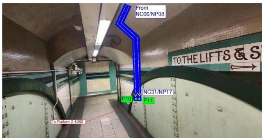
Figures 10 & 11: Proposed new cabling in the stairways and passages of the station. Proposed new CMS shown in blue. The CMS will be colour matched to the surface which it sits on.
