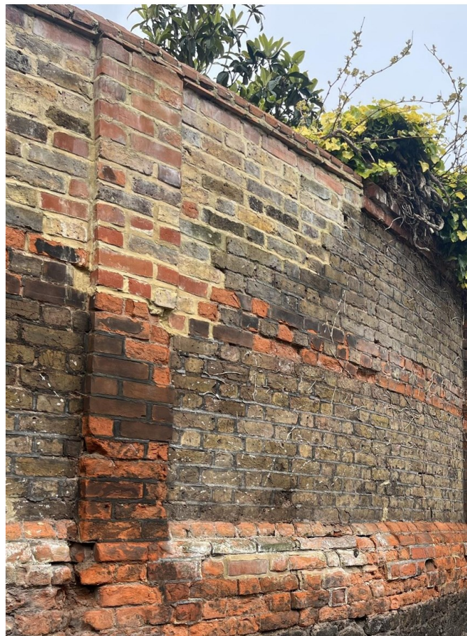
Section of rebuilt wall of low quality
