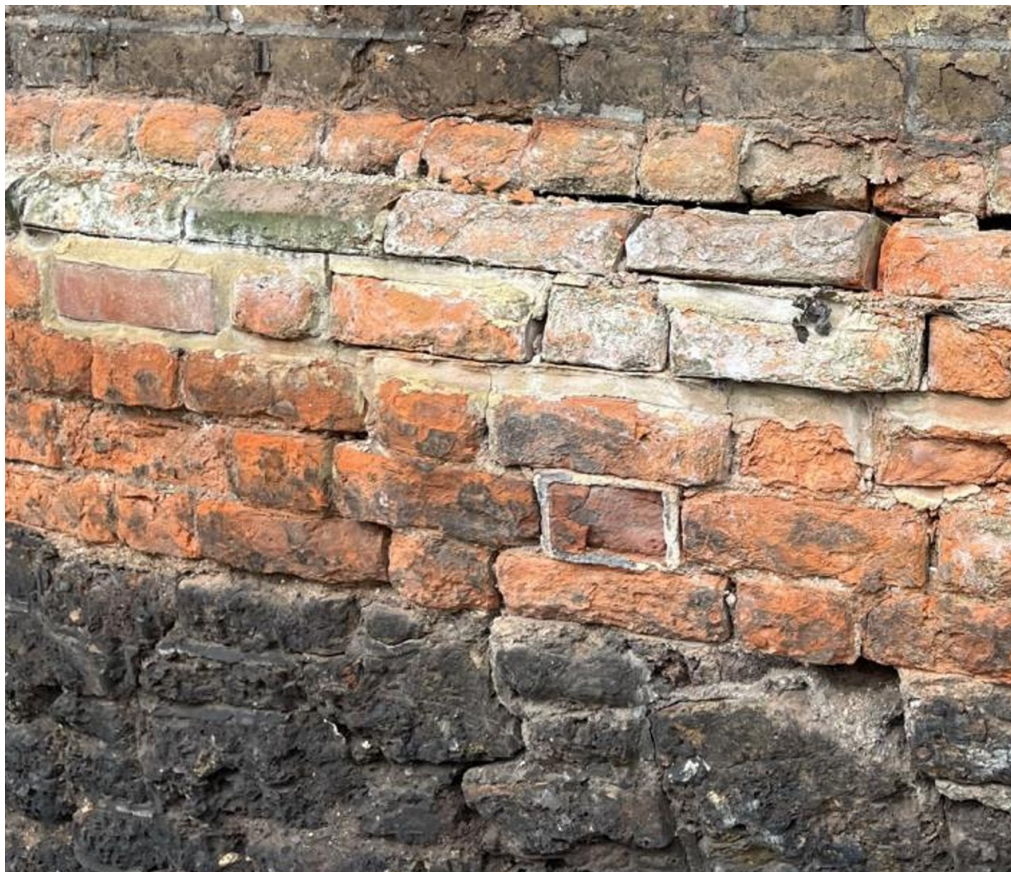
Example of eroded soft red brick, washed joints and low quality cement pointing.
