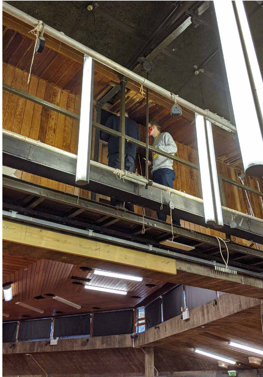
The ceiling void is accessed via a gantry above the stage.
