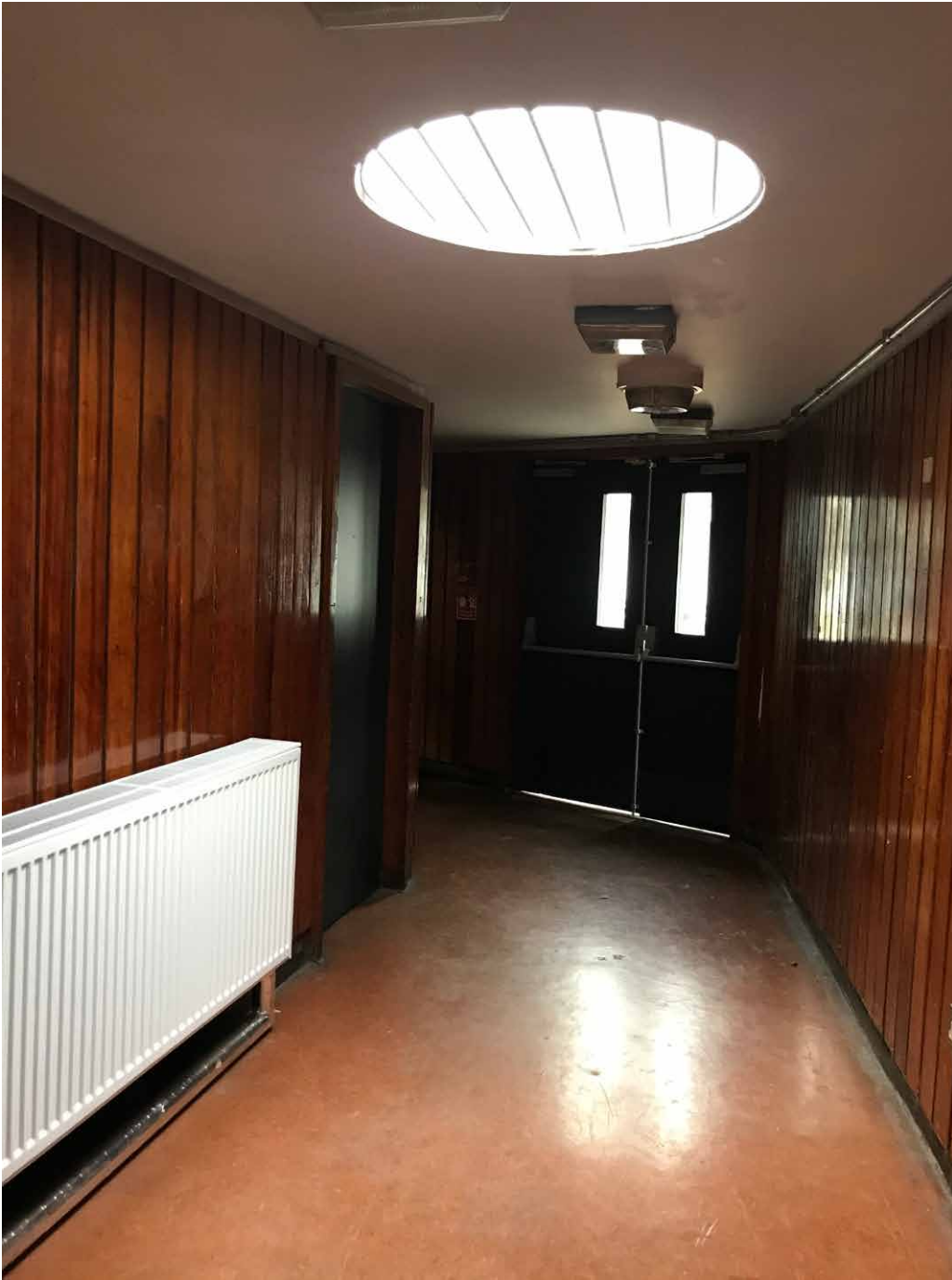
A single colour sheet flooring remains in part of the corridor. It is not known whether this is the existing floor. Radiators in the corridor are less appropriate for the building than those recently installed in the main hall. The foil lagging is also visually insensitive.
