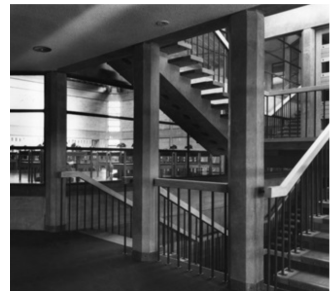
Chamfered concrete columns. Main Staircase. University Centre, Cambridge
