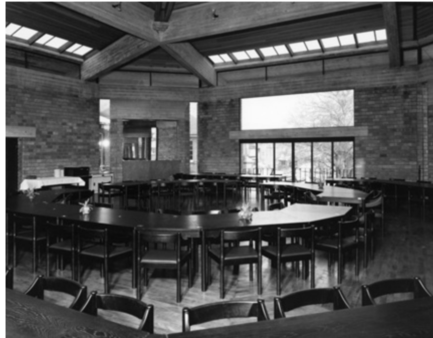
Board-marked concrete and timber boarded ceiling, Dining Hall, Darwin College Cambridge
