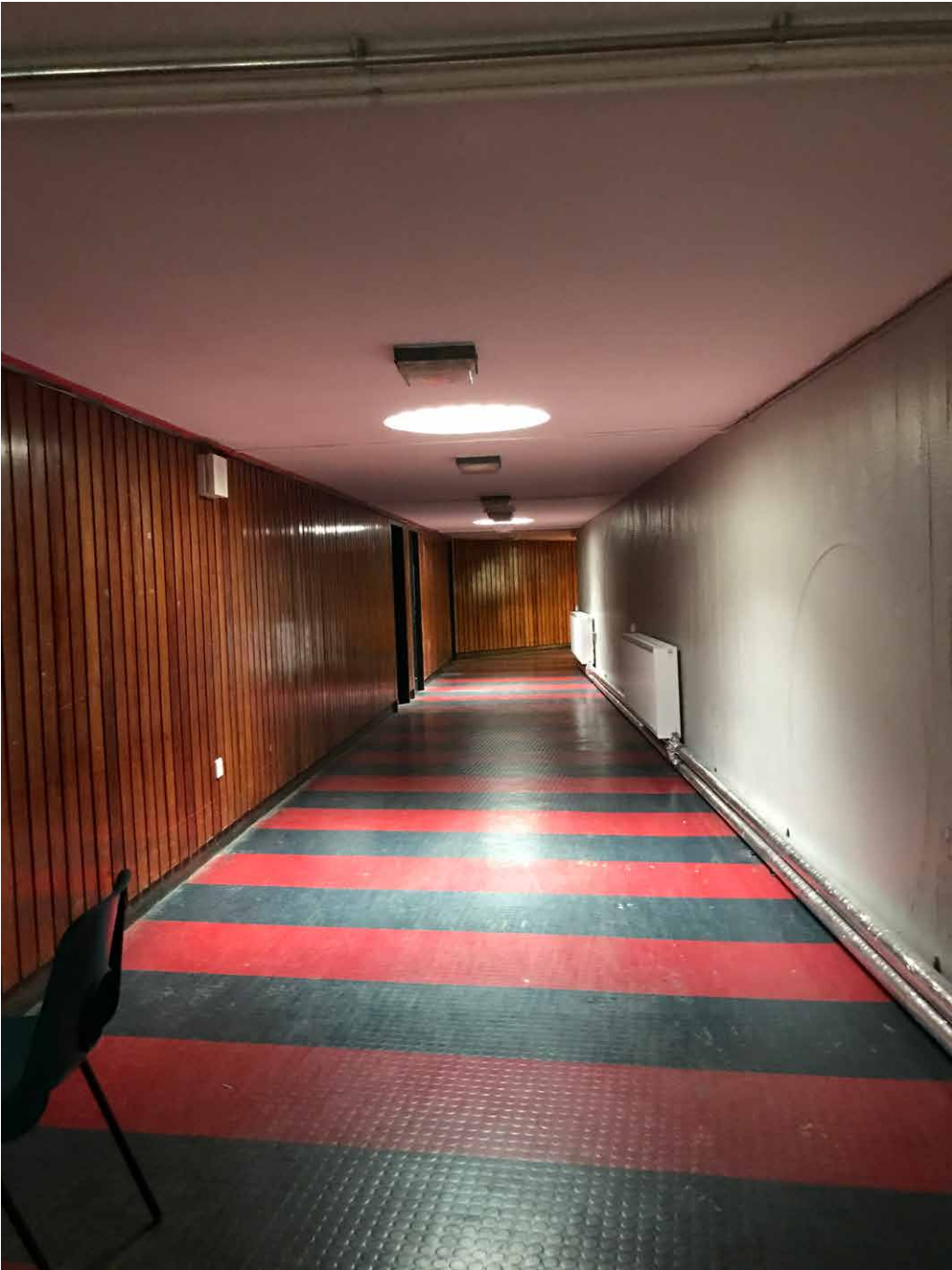
The original flooring to the corridor has been replaced, and the striped, studded rubber current flooring pictured above installed prior to the building's listing. The original concrete has been painted to one side of the corridor and ceiling, and new bulkhead light fittings installed. The outline of infilled circular holes is visible to the right hand side of the image.
