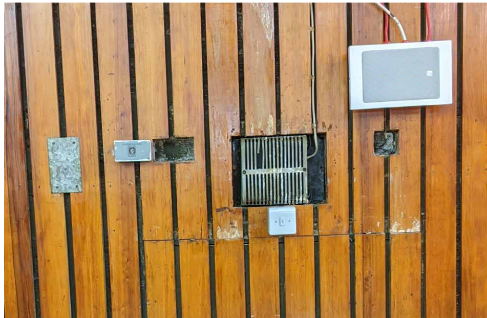
In general, redundant services installations remain in place, and have damaged small but numerous areas of the timber lining.
