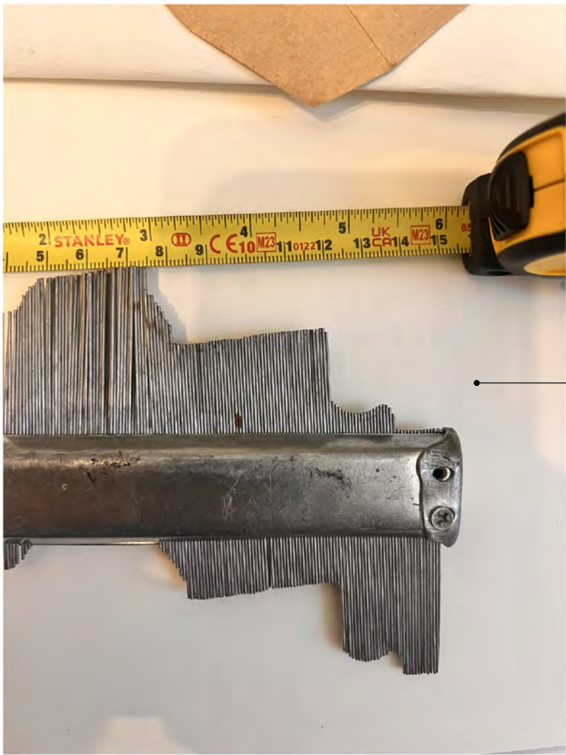
02: EXISTING WINDOW W.2.6 EDGE PROFILE SCALE N/A
