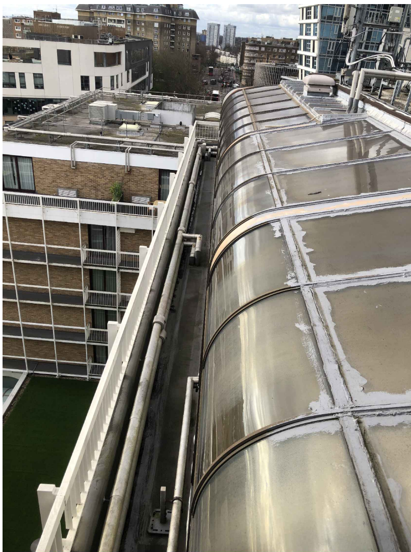
Discolouration & repairs to glazing panels
