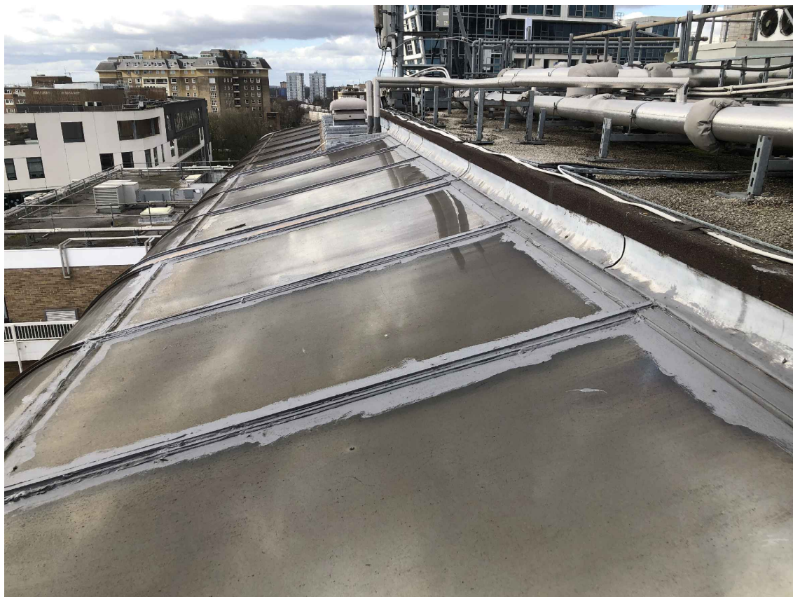
Liquid membrane repairs
