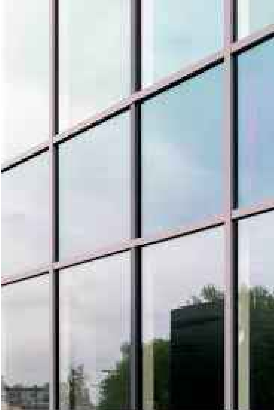
Contemporary 'stick frame' assembly replacement curtain wall system using 50mm mullions and transoms (appearance to match existing).
