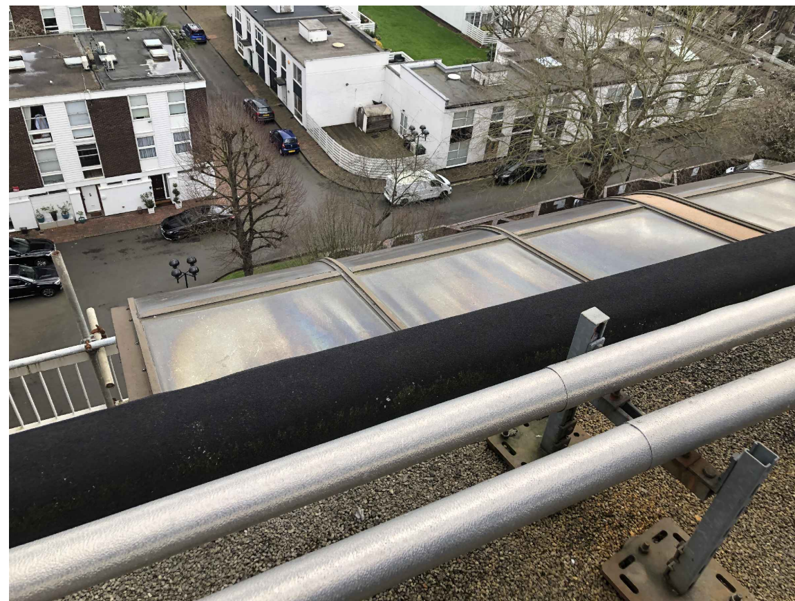
Discolouration to glazing panels
