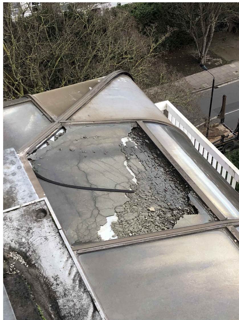
Impact damage to glazing panel
