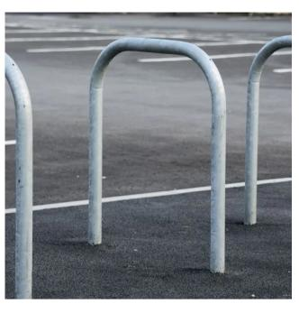
715mm W x 800mm H Proprietary Sheffield cycle stand as shown to area of East facing elevation
