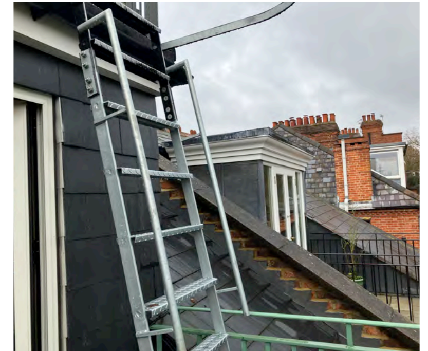
Access ladder to dormer roof
