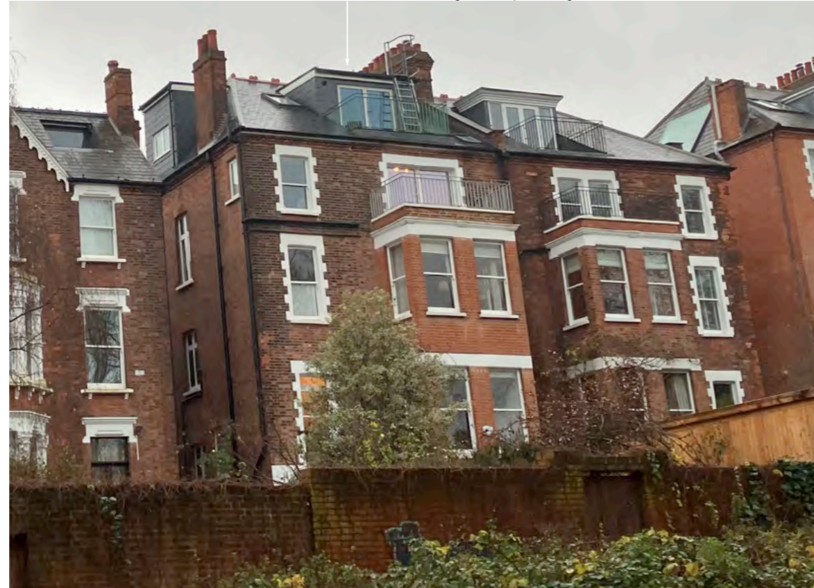
17 Tanza Road (Left) and 19 Tanza Road (Right) from the rear of the properties
