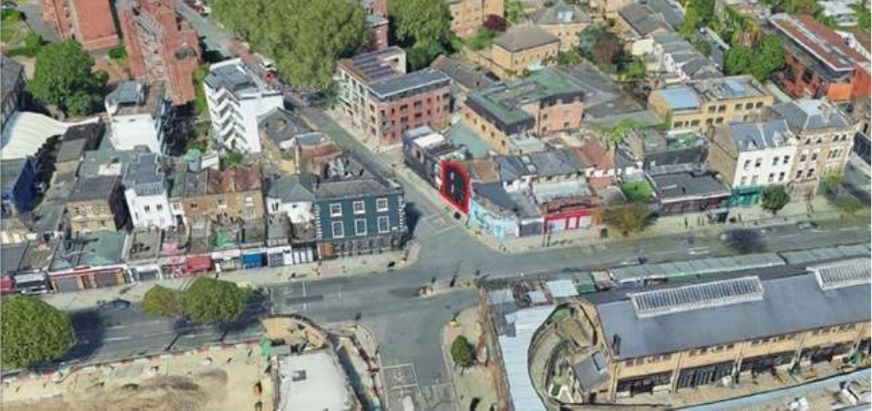
Figure 2 - Aerial images of the site
