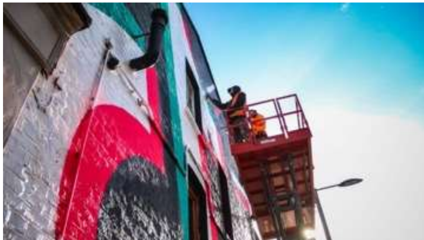
Figure 7 - Use of scissor lift in accordance with highways permit
