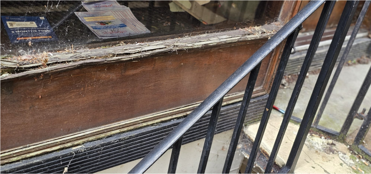
53a Marchmont Street - Photo 2-3-4
