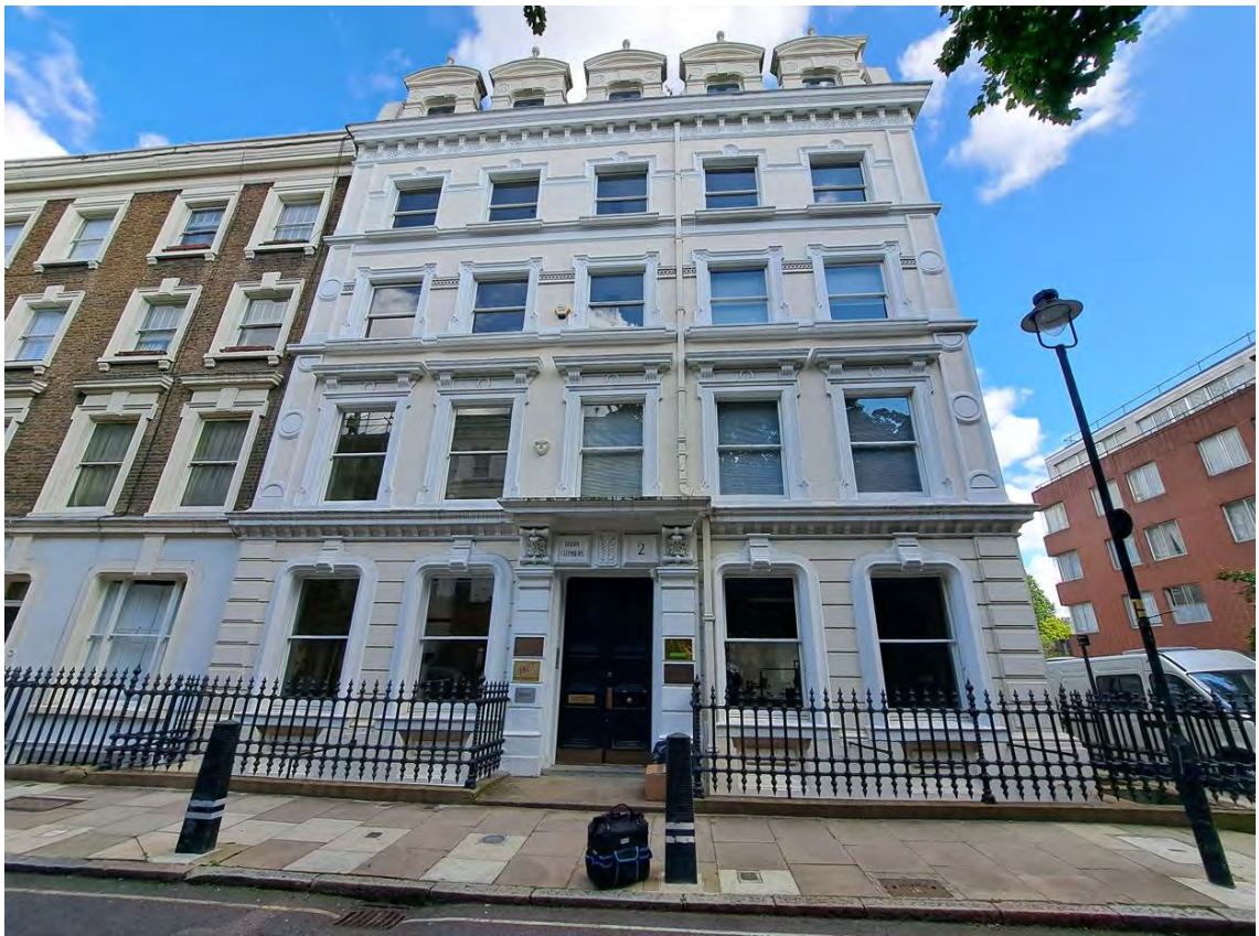
Photo 01: Southern side of the building and main entrance.
