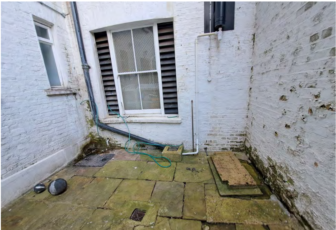
Photo 08: Lower ground floor outdoor courtyard.
