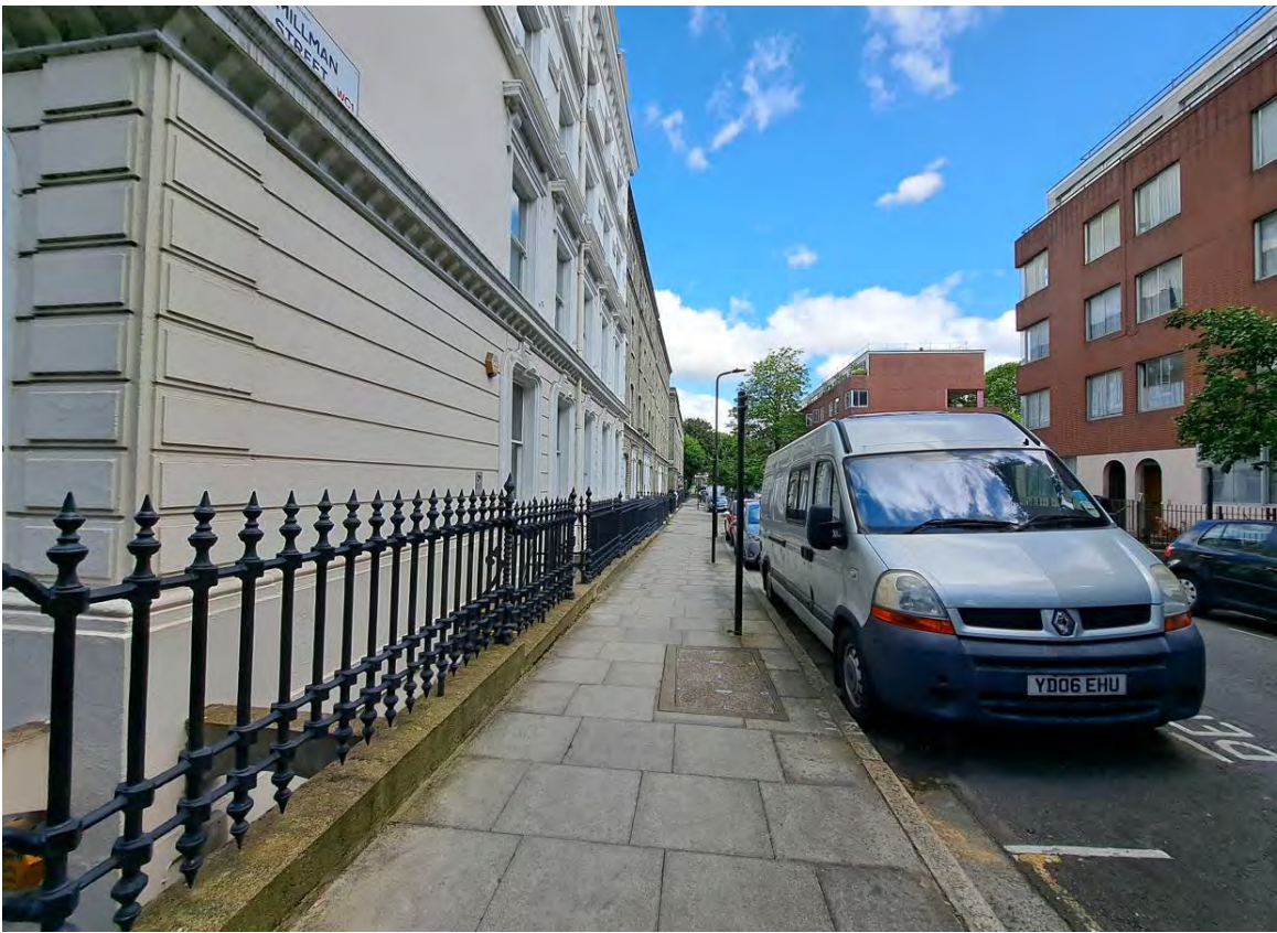
Photo 03: Eastern side of the building.
