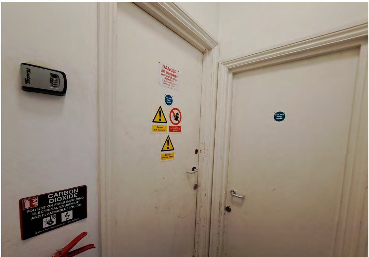
Photo 05: Lift maintenance room and boiler room on lower ground floor.
