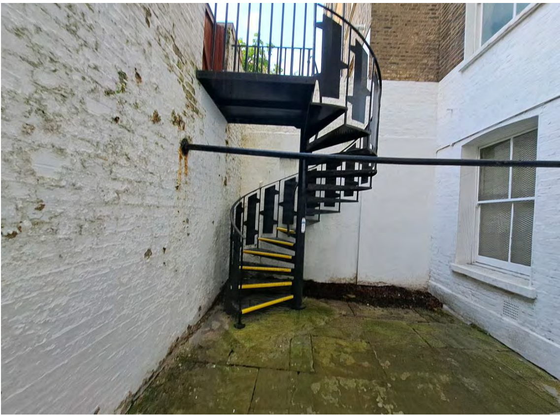
Photo 07: Lower ground floor outdoor courtyard.
