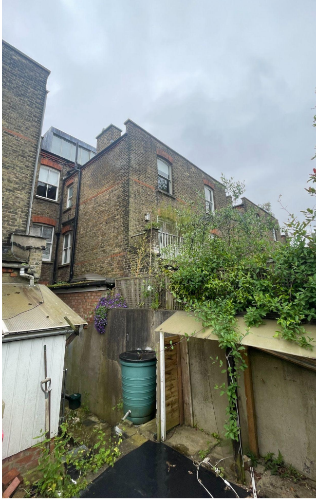
Constantine Road rear existing extension and view of the 07 property
