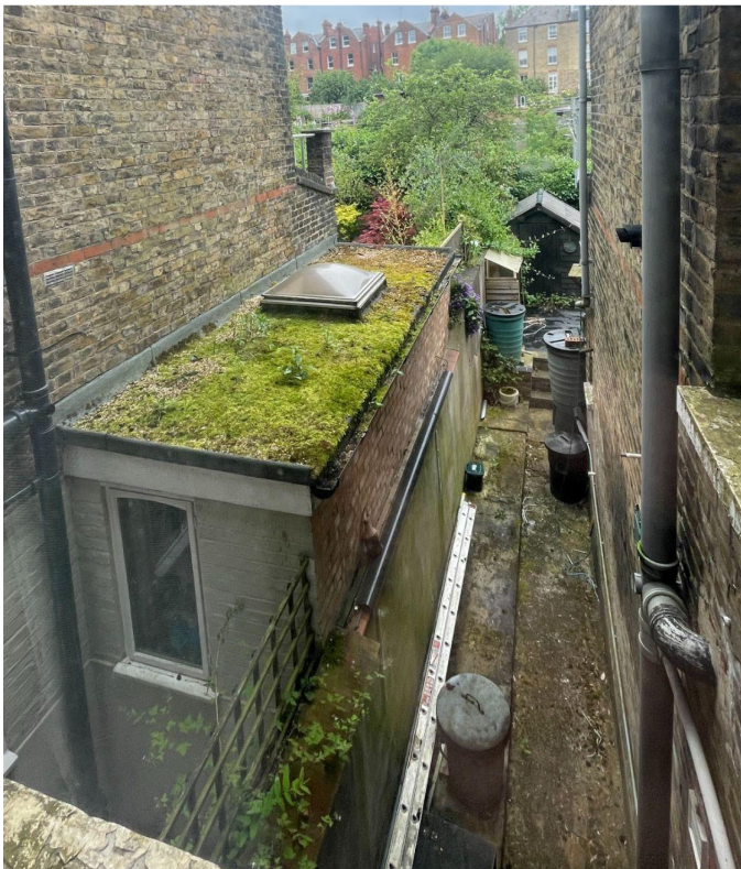
Constantine Road site view of the neighbour's existing side extension
