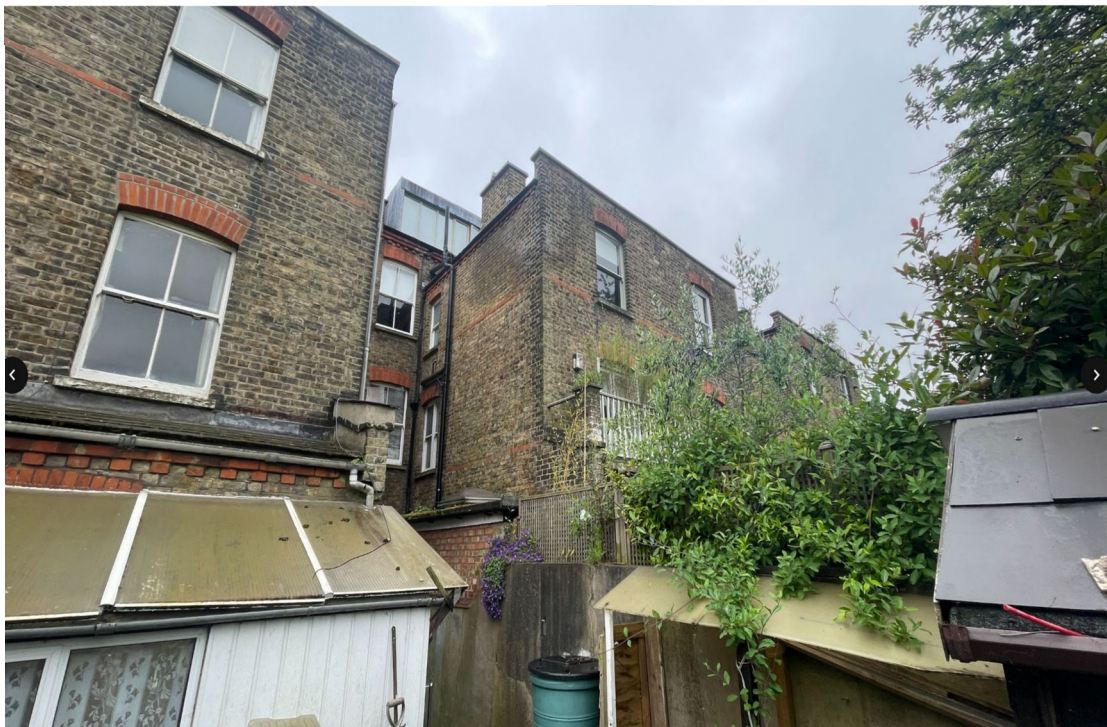
Constantine Road rear existing extension and view of the 07 property
