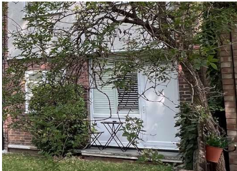
Figure 4 - 161 Goldhurst Terrace window 1 and 2 are numbered left to right.
