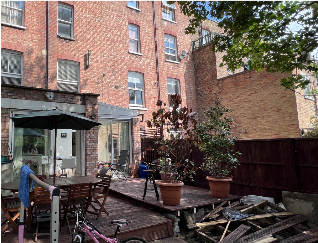
View of existing extension in relation to extension at 155 Goldhurst Terrace
