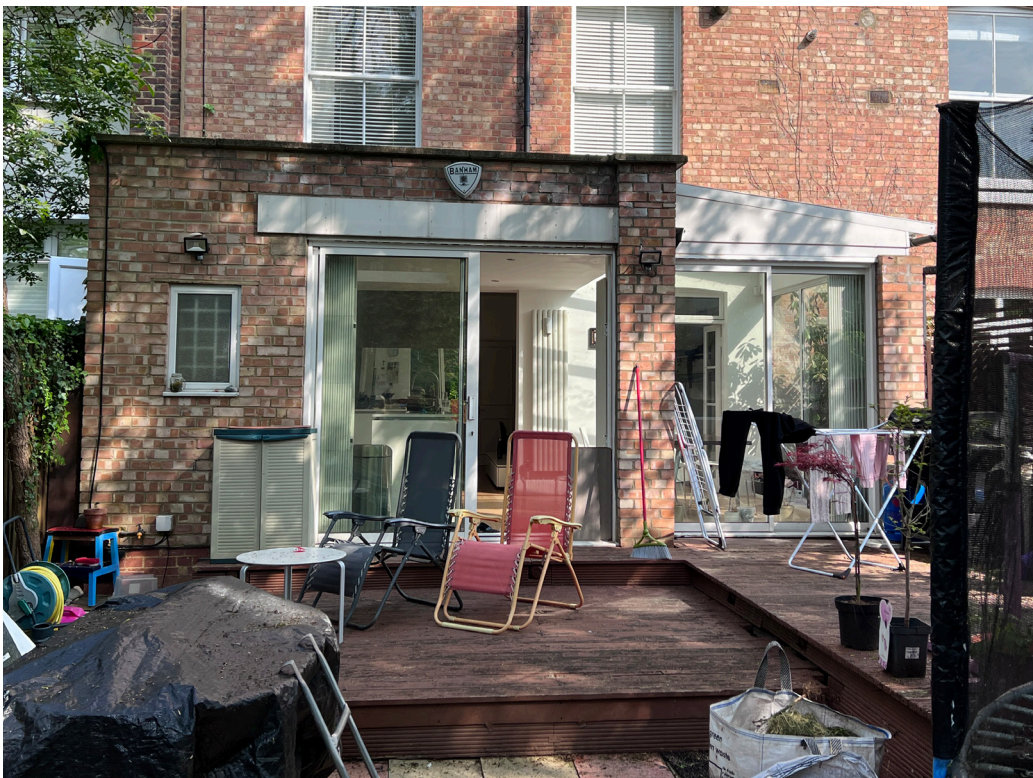
Rear view of existing extension
