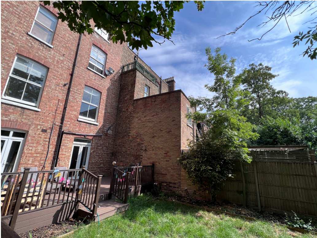
Garden to 157 Goldhurst Terrace towards rear extension at 155 Goldhurst Terrace
