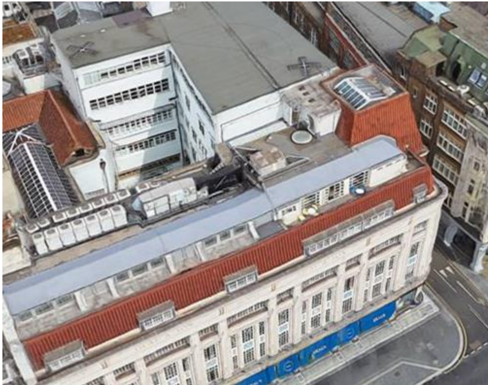
Figure 2.3: Roof of Heals building today (image provided by google maps)
