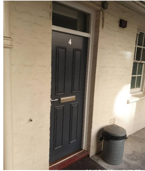
REPLACED: Flat 4 Front Entrance Door
