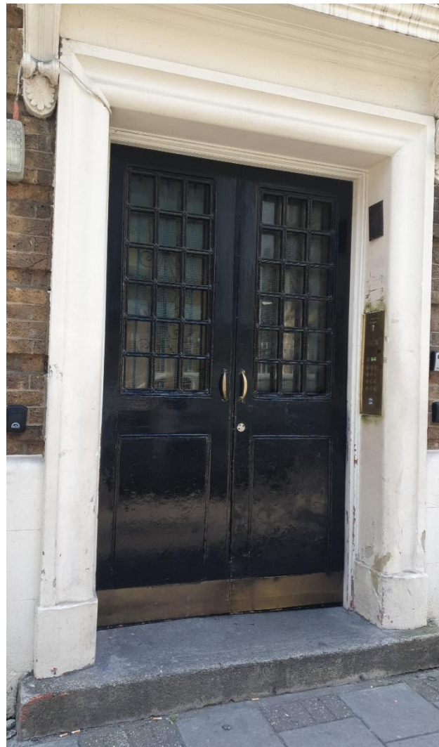
Photo 15: Communal Front Entrance Door (not being replaced)
