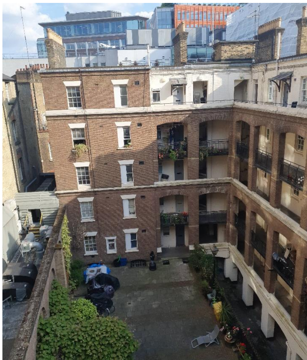
Photo 9: Viewing South towards Block (Streatham Street behind)
