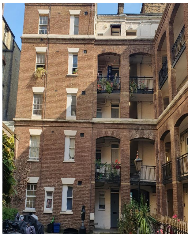
Photo 2: Facing south towards Streatham Street from Courtyard
