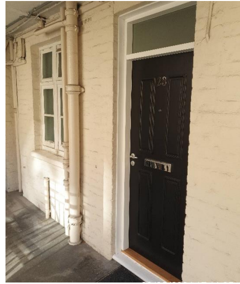
REPLACED: Flat 28 Front Entrance Door
