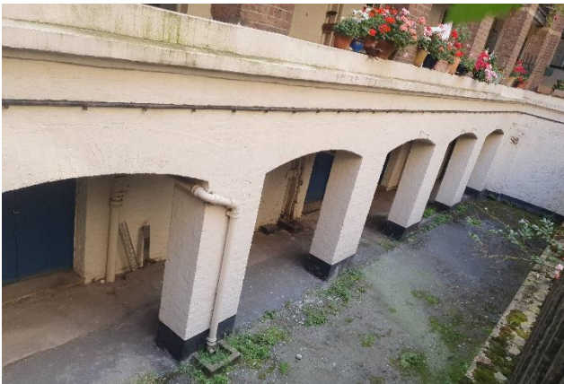
Photo 13: Viewing West basement level from ground floor Courtyard
