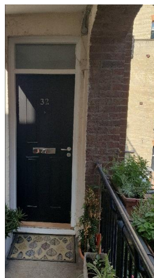
REPLACED: Flat 32 Front Entrance Door
