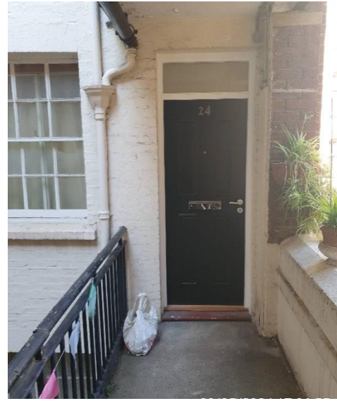
REPLACED: Flat 24 Front Entrance Door
