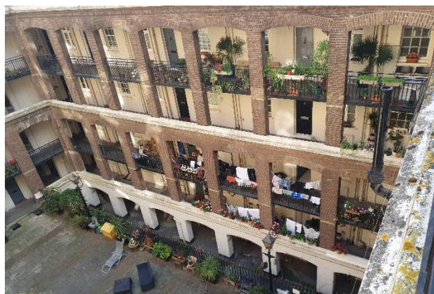
Photo 12: Viewing West towards Main Block from top floor (Dyott Street behind)
