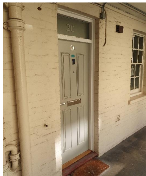
REPLACED: Flat 20 Front Entrance Door
