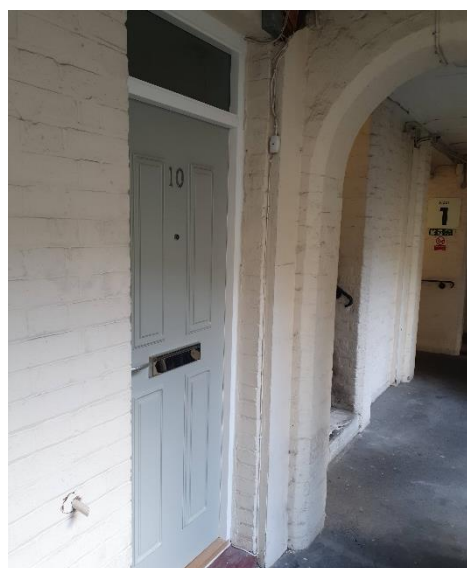
REPLACED: Flat 10 Front Entrance Door
