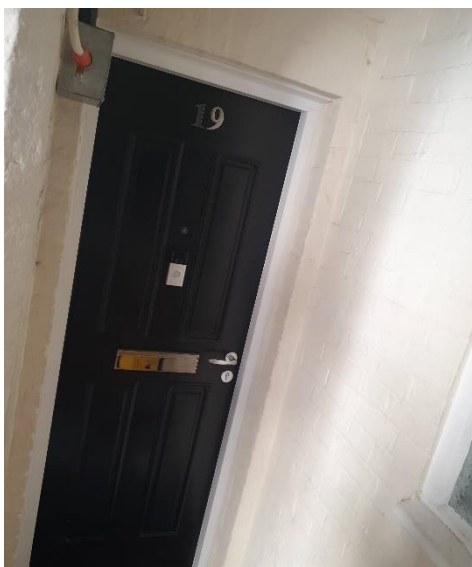
REPLACED: Flat 19 Front Entrance Door
