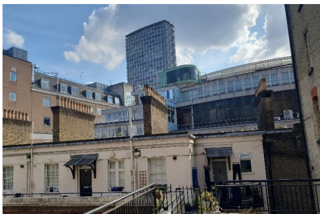
Photo 11: Viewing West towards Top floor corner (Dyott Street behind)
