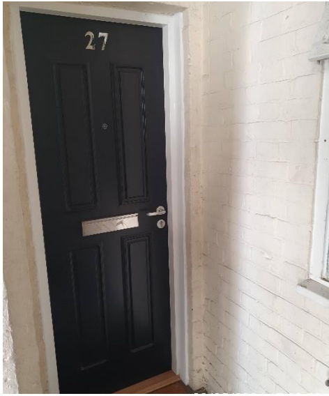
REPLACED: Flat 27 Front Entrance Door
