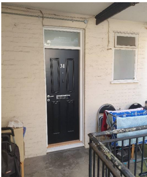
REPLACED: Flat 31 Front Entrance Door
