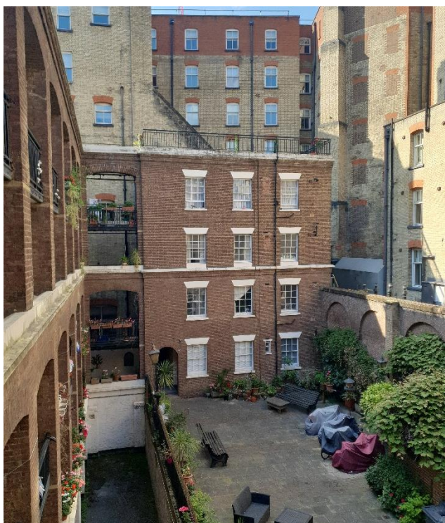
Photo 7: Viewing North towards Flats 8, 16, 24, and 32
