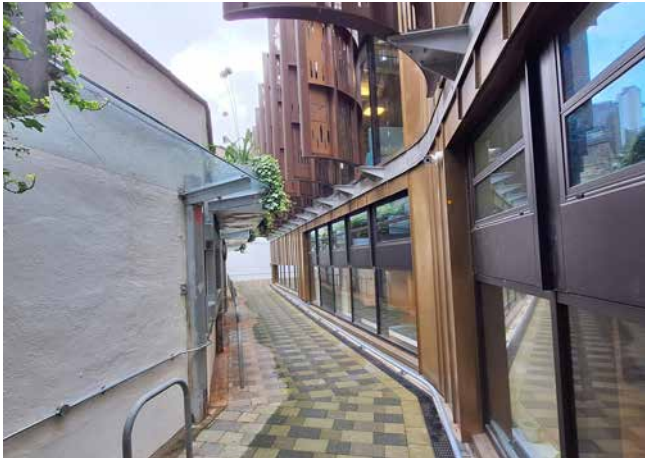
Fig 04: Eastern view of external access area.
