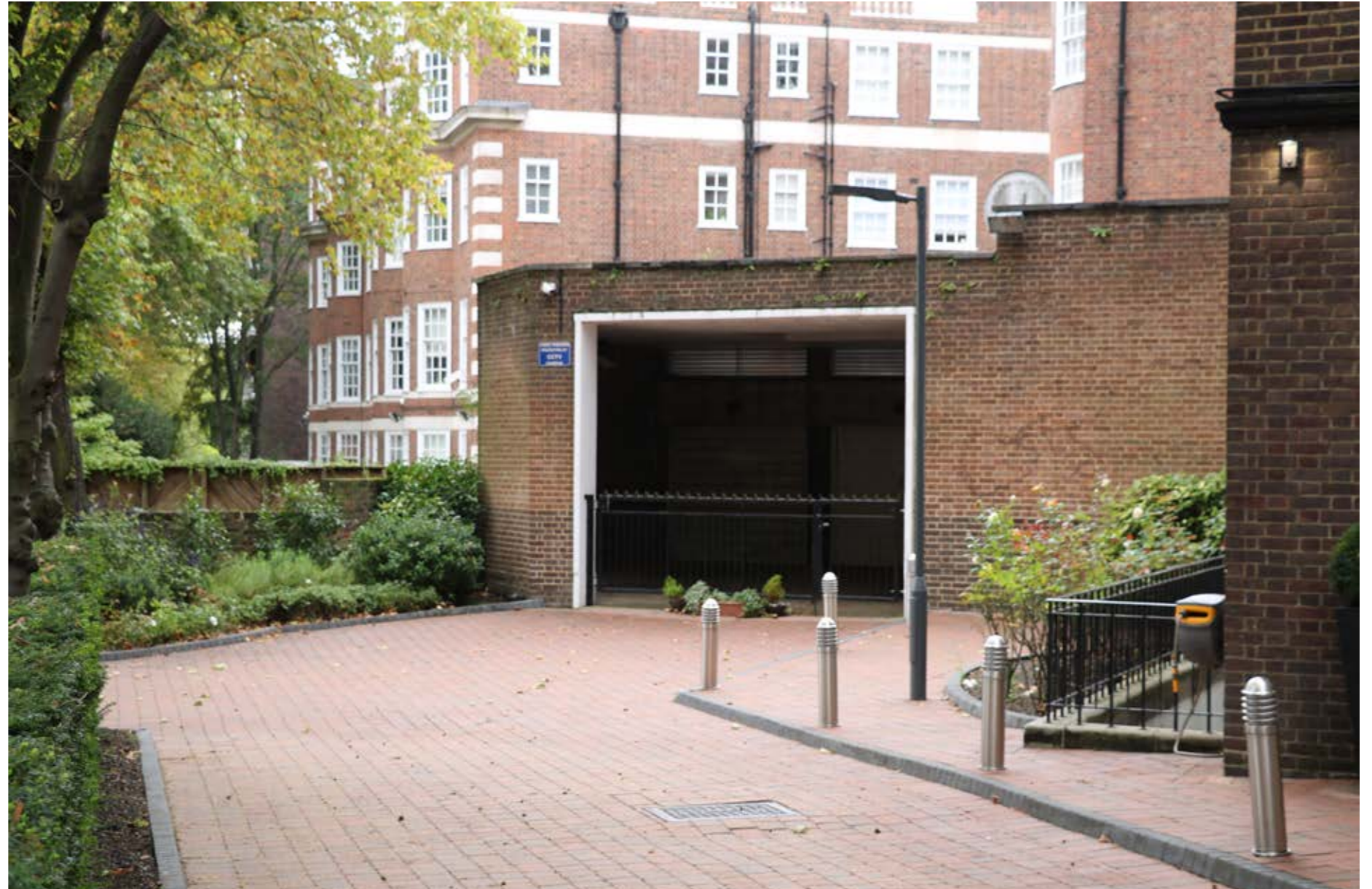
Fig 15. View of the existing garage from within the forecourt / front driveway area with the disused garage doorway in-filled with railings.
