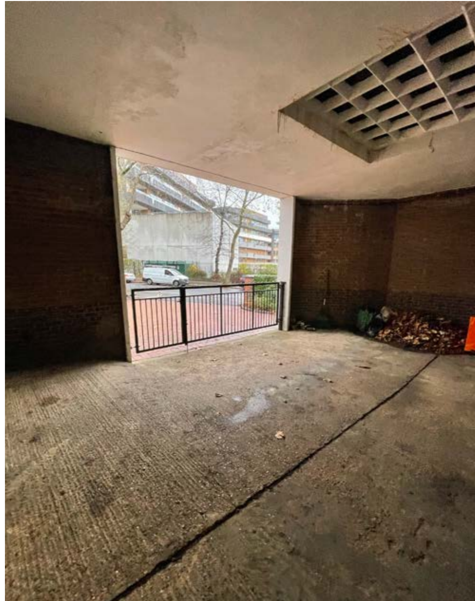
Fig 19. View from within the existing garage looking out towards Avenue Road.
