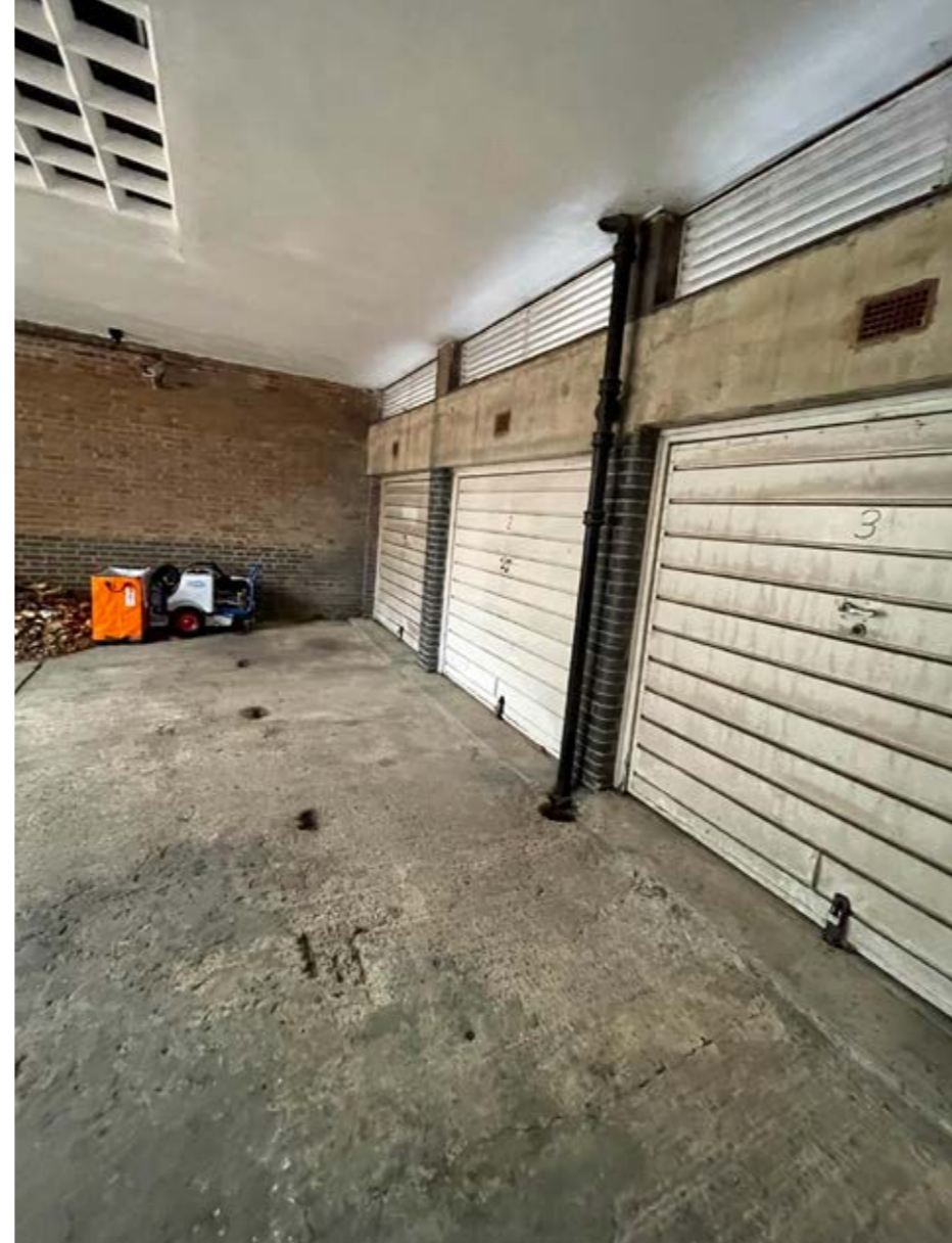
Fig 20. The existing lock-up garages within the garage enclosure.
