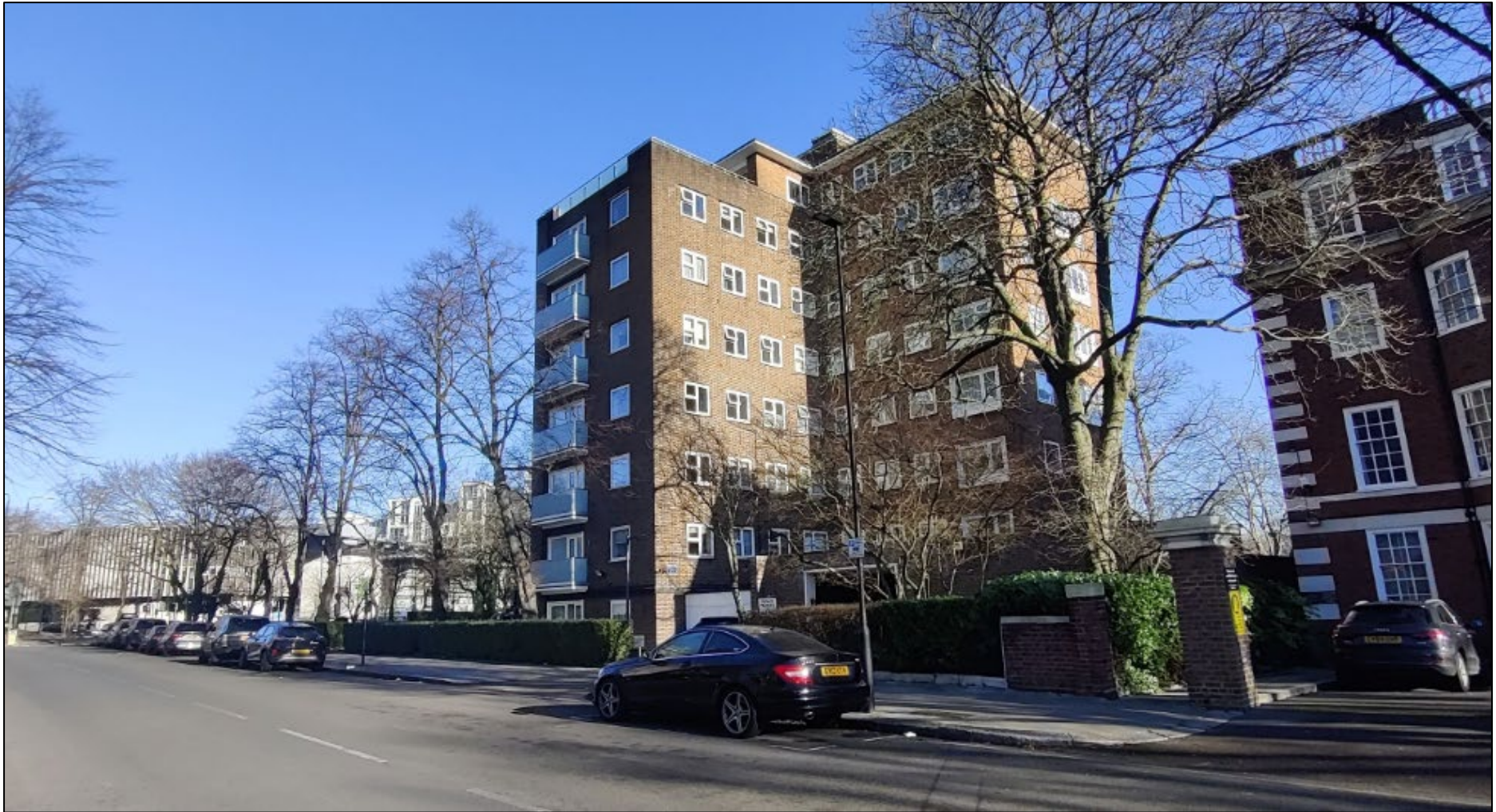
Photograph 2: 95 Avenue Road viewed from St Johns Wood Park
