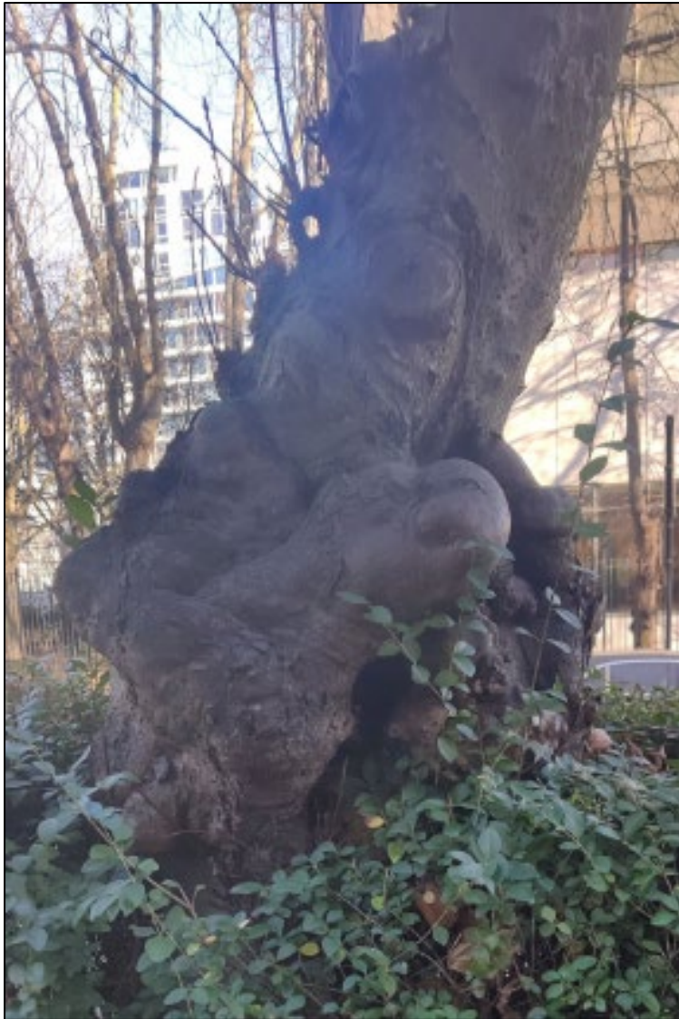
Photograph 3: Cavity in base of T6
