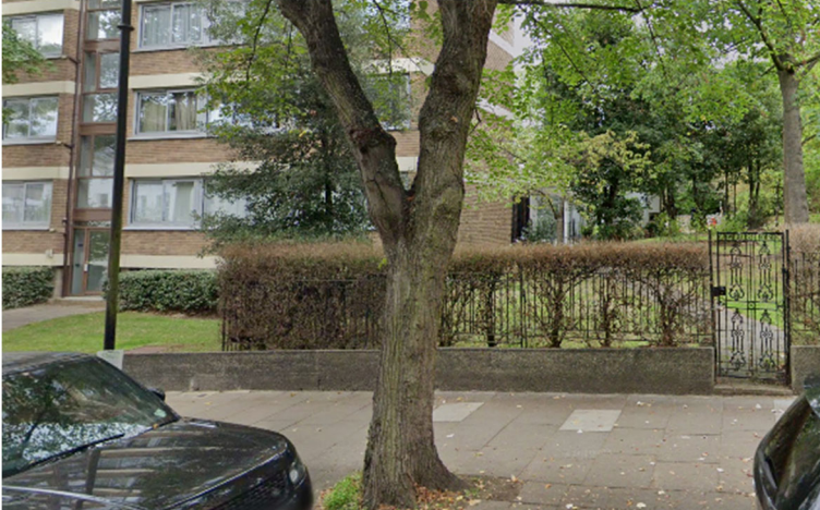
Fig 7_View of existing concrete wall and existing railing from St Edmunds Terrace.
