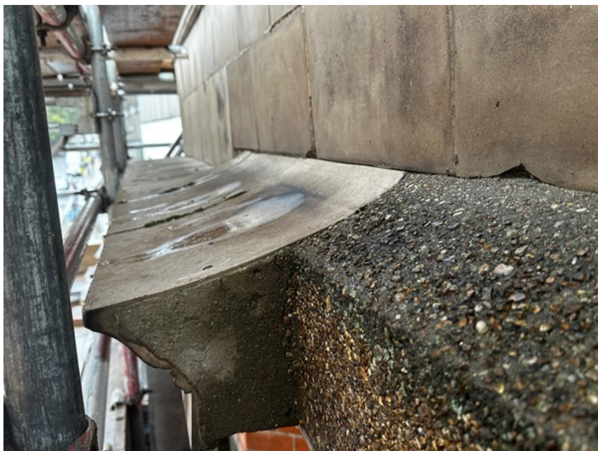
Figures 5 and 6. A view of a terracotta console where the front section has broken away. Cracking extends across the full length of the console. Note, terracotta soffit tiles at the front of the balcony have been replaced with a cement render. The image below shows a section of original terracotta cornice surviving at the left hand (south) end.
