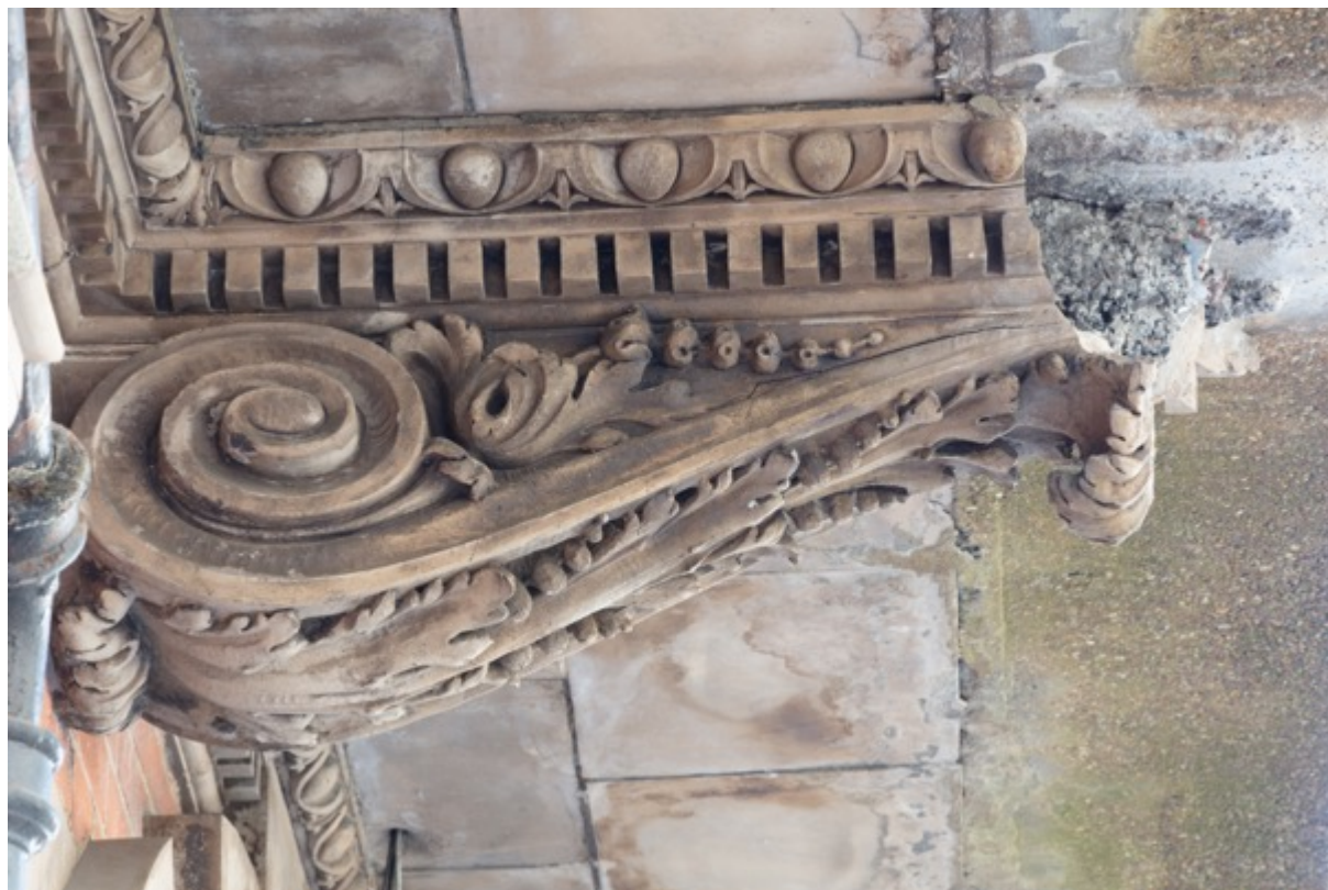
Figures 5 and 6. A view of a terracotta console where the front section has broken away. Cracking extends across the full length of the console. Note, terracotta soffit tiles at the front of the balcony have been replaced with a cement render. The image below shows a section of original terracotta cornice surviving at the left hand (south) end.
