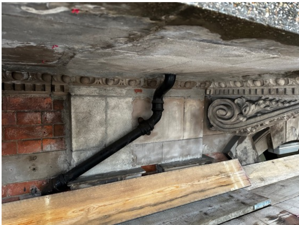
Figures 9 and 10. Two areas of ashlar terracotta below the balcony which have been crudely replaced with cement render. This work appears to relate to alterations to the rainwater drainage.
