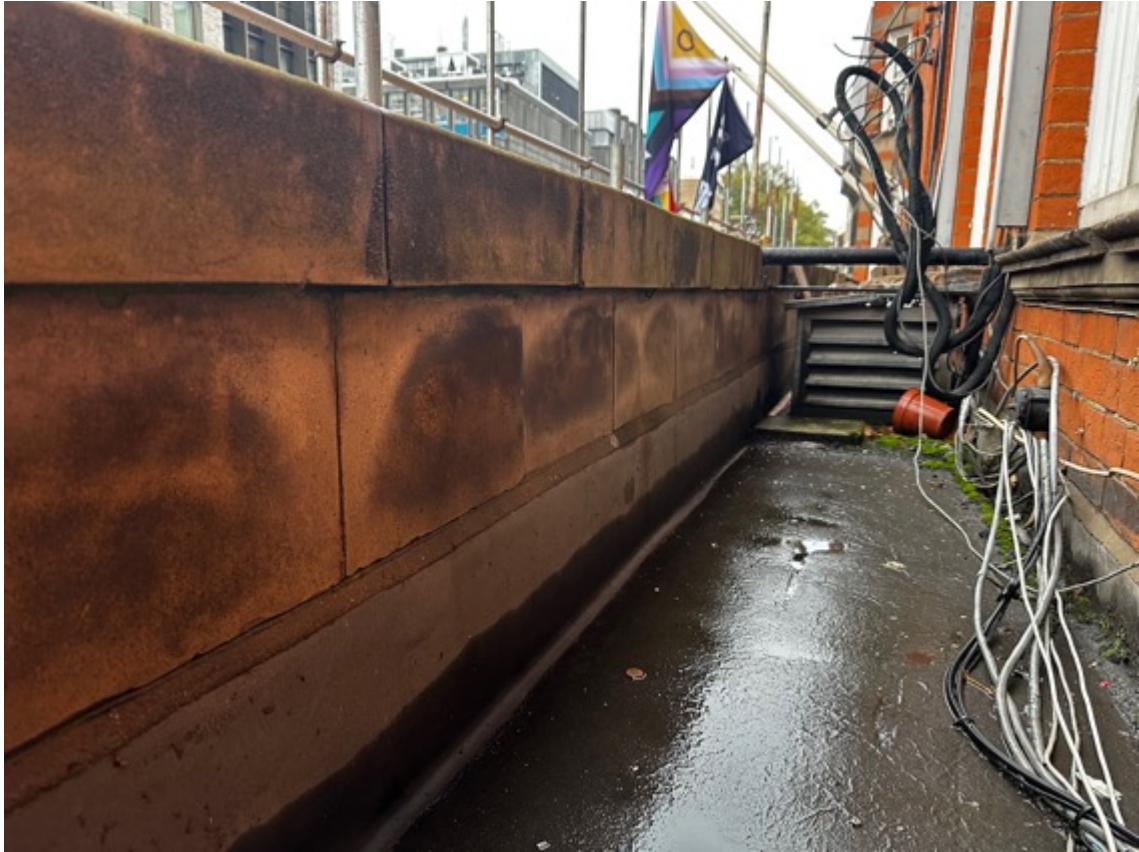
Figures 11 and 12. The existing mastic asphalt. Cracks, splits and bulges are present. One of the two existing cast iron rainwater outlets. The internal dimension is only 44mm and there is very little drainage fall towards the outlets
