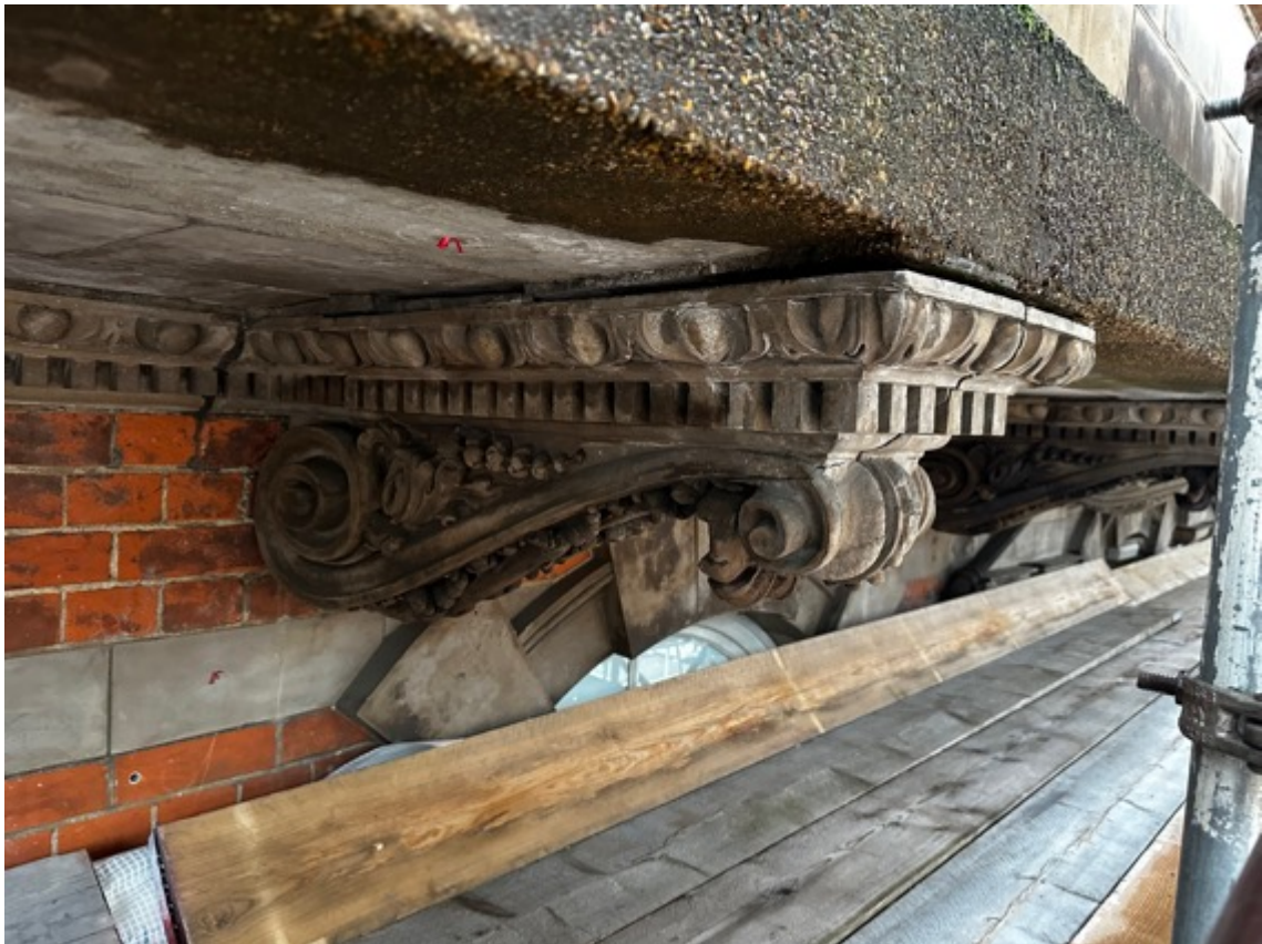
Figures 3 and 4. Expansive corrosion of the steel balcony support and expansion of the saturated clinker concrete within the terracotta console has caused extensive cracking and failure. The image below shows the missing terracotta cornice which has been replaced with a crude exposed aggregate concrete repair.
