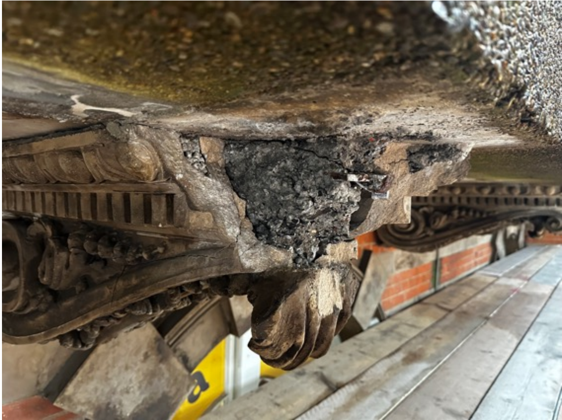
Figures 3 and 4. Expansive corrosion of the steel balcony support and expansion of the saturated clinker concrete within the terracotta console has caused extensive cracking and failure. The image below shows the missing terracotta cornice which has been replaced with a crude exposed aggregate concrete repair.
