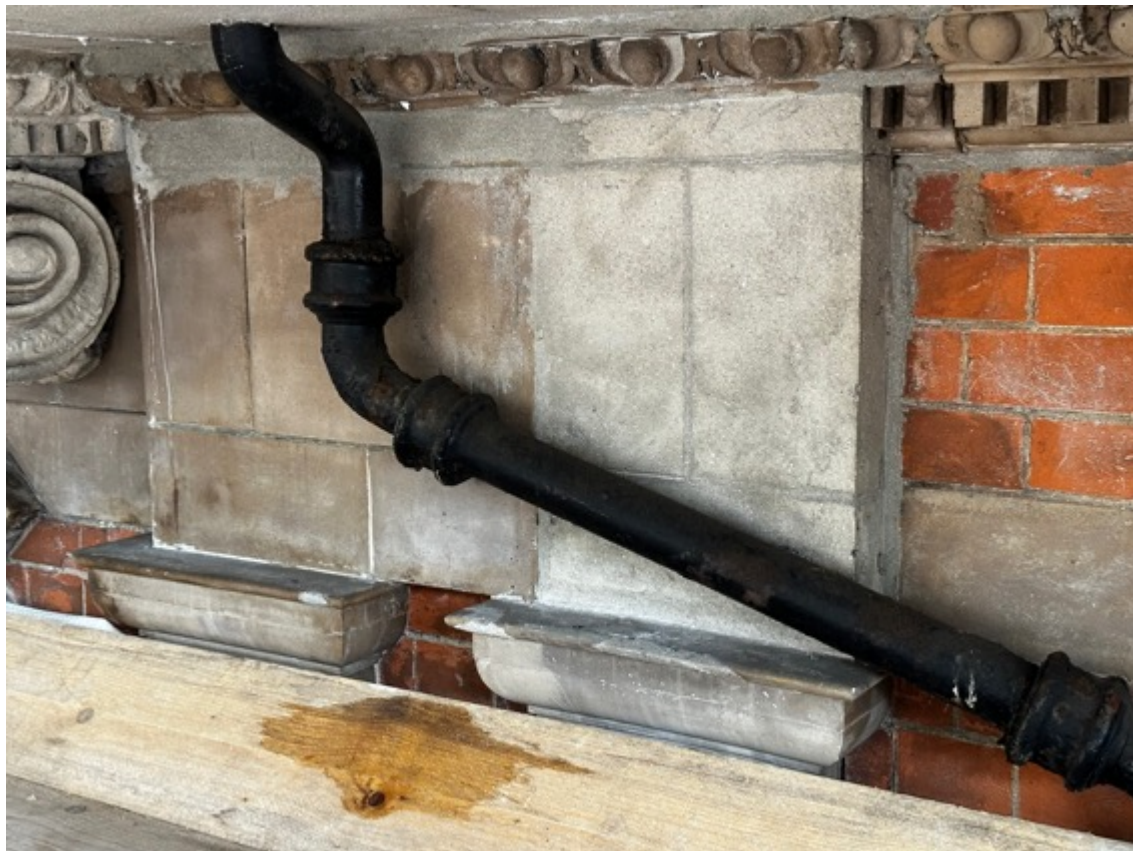
Figures 9 and 10. Two areas of ashlar terracotta below the balcony which have been crudely replaced with cement render. This work appears to relate to alterations to the rainwater drainage.
