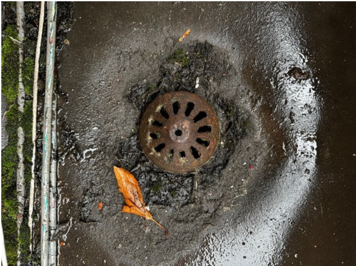
Figures 11 and 12. The existing mastic asphalt. Cracks, splits and bulges are present. One of the two existing cast iron rainwater outlets. The internal dimension is only 44mm and there is very little drainage fall towards the outlets
