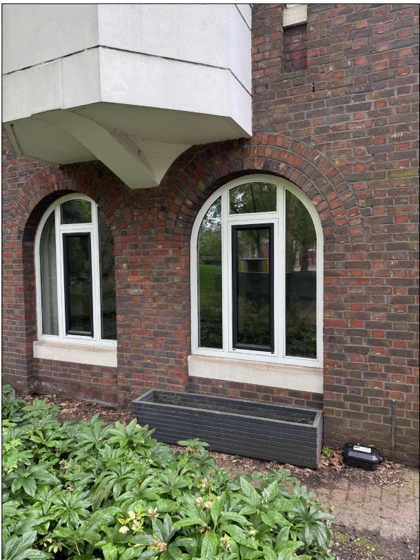
5. Existing Building- Windows W001 & W002
