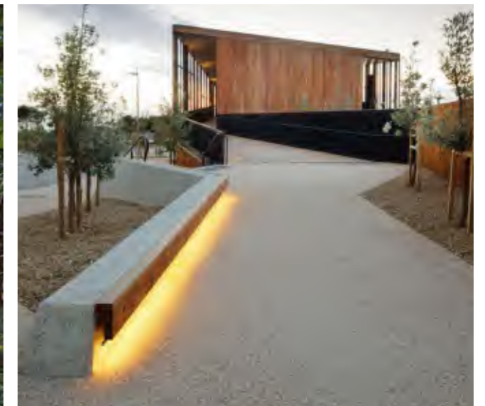
Integrated balustrade lighting
