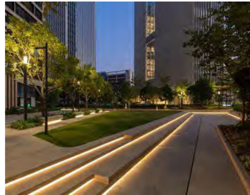
Functional and accent landscape lighting for terrace area
