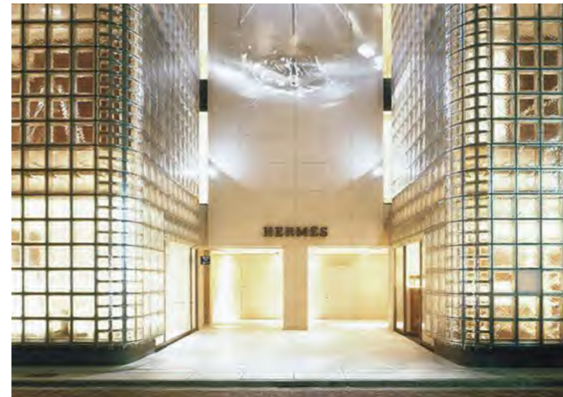
Illuminating the façade from the interior
