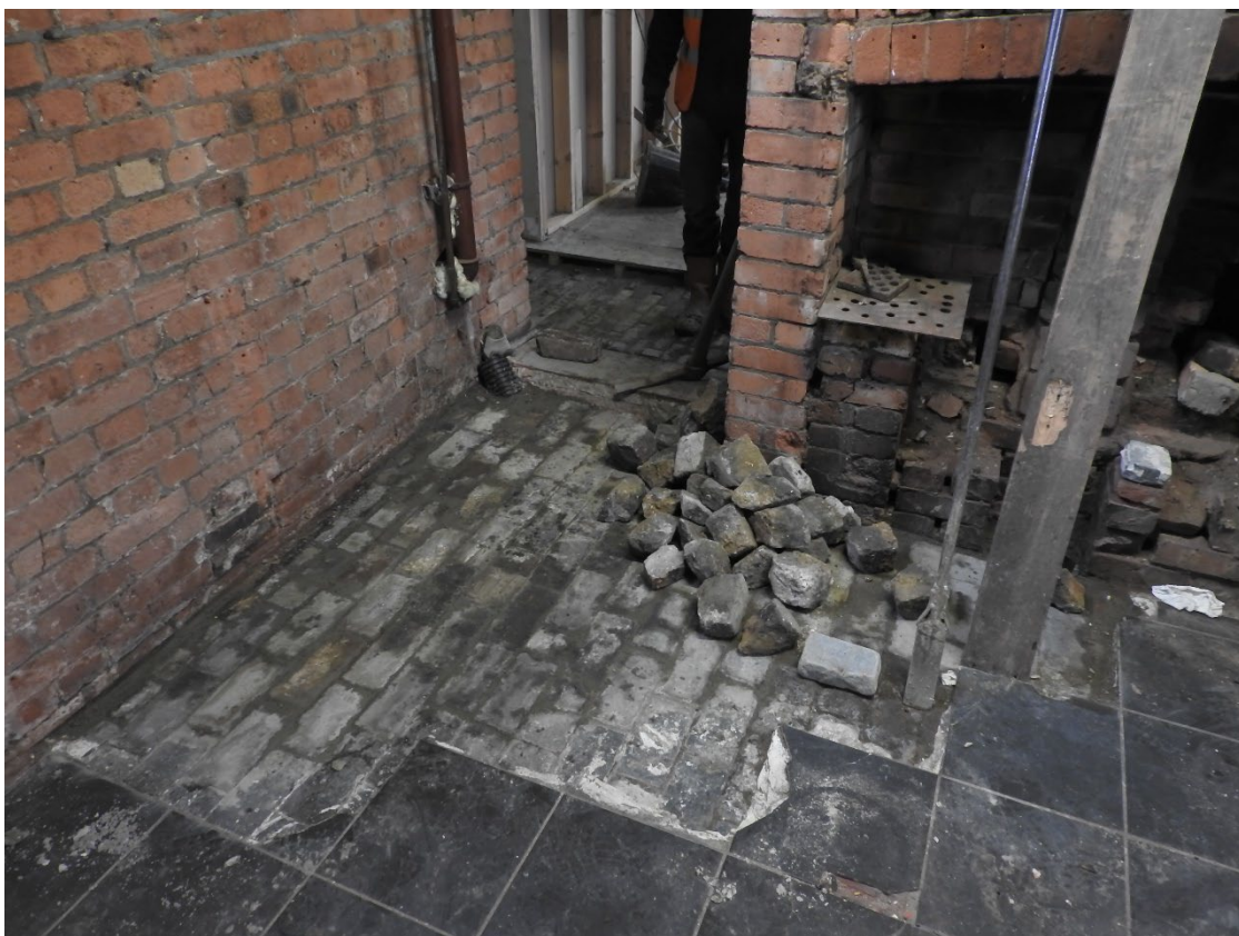
Removal of tiles and repairs to original floor
