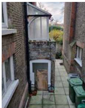
Existing Side passage views
