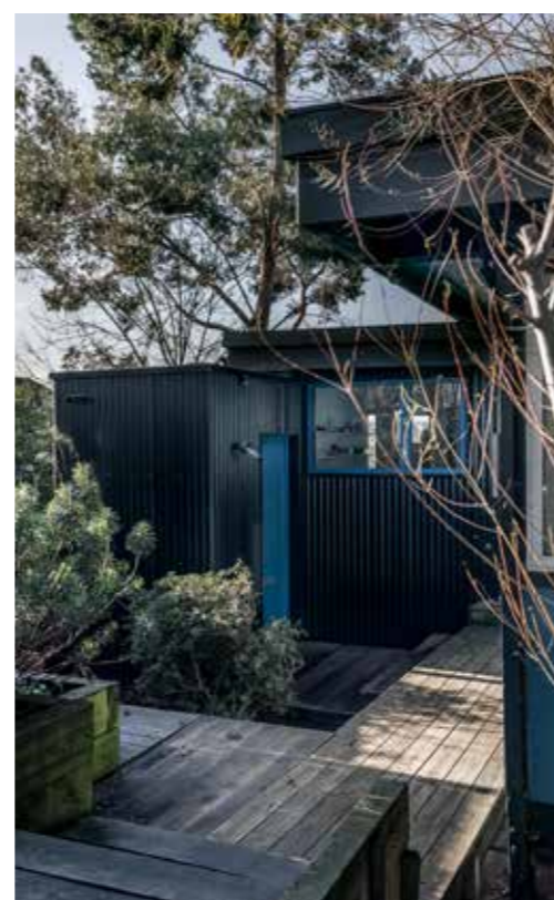
Extension and alterations to Segal House, Lewisham
