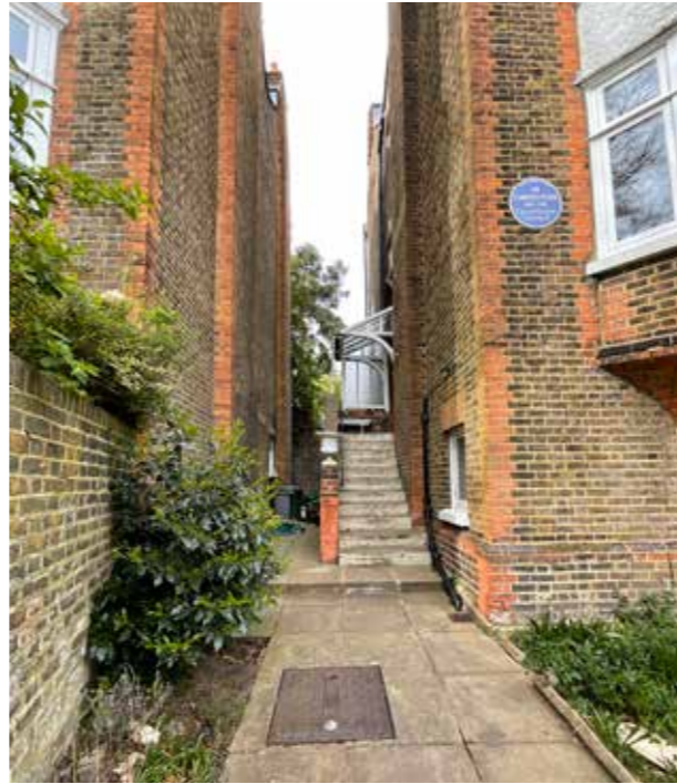
Entrance stair and canopy
