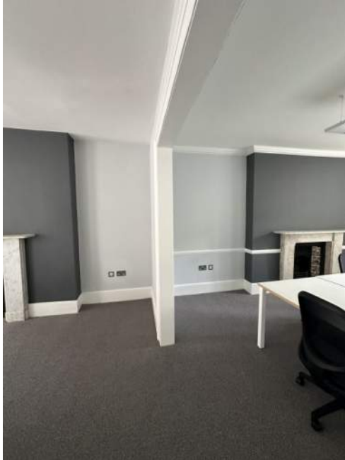
Figure 17: The modern opening in the spine wall at 2 nd floor level.
