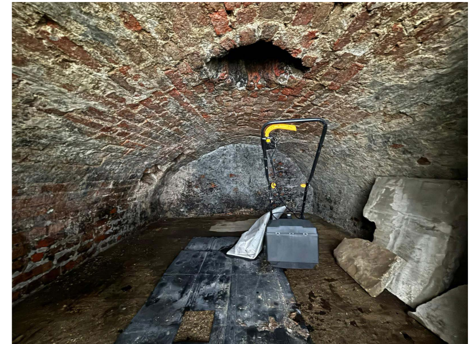
Existing front cellar vaults
