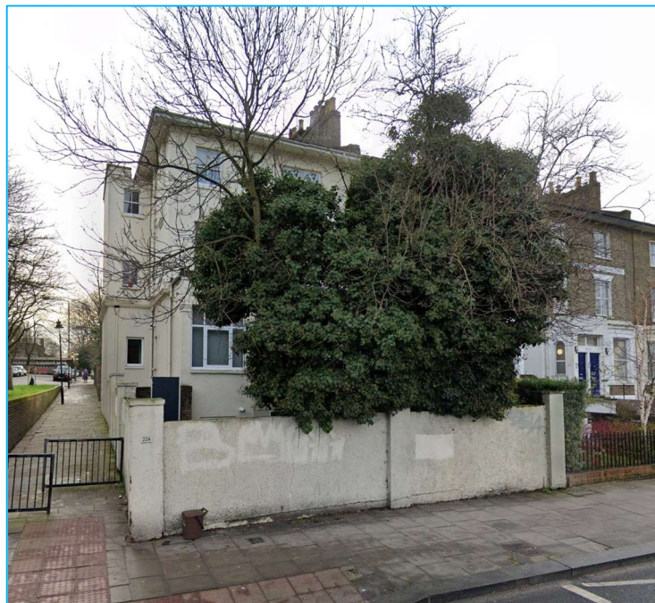
No. 226 has a wall to the front and its configuration does not resemble its neighbours from the street scene
