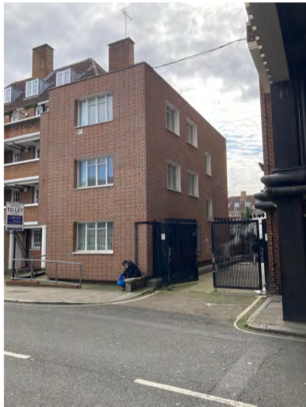
EXISTING SECURE GATING TO ACCESS ROAD LEADING TO PROPOSED CYCLE STORE SITE.
