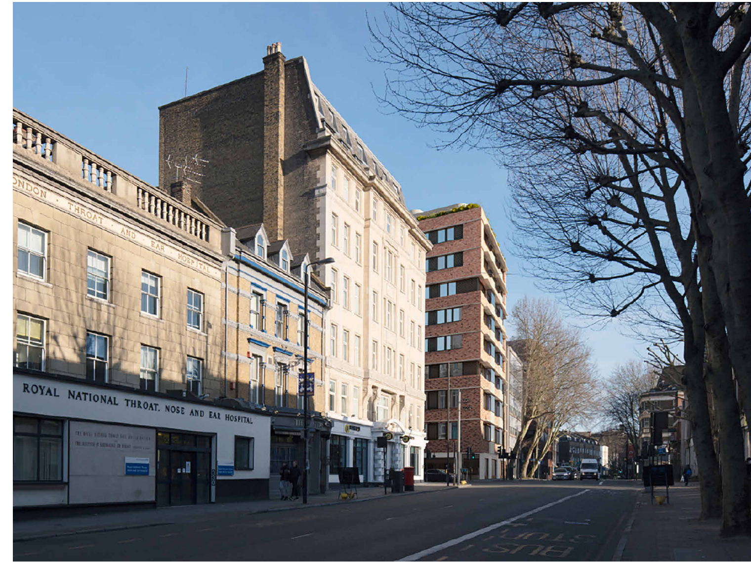
CGI with Plant in Red - Not Visible in View Gray's Inn Road (North)
