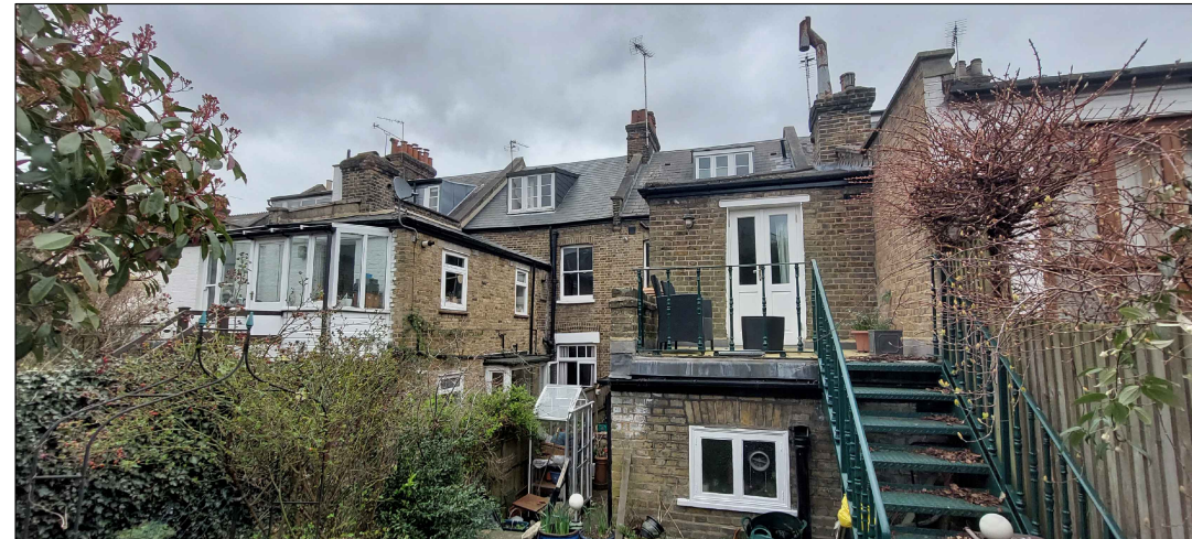
View of rear elevation (taken 2023)
