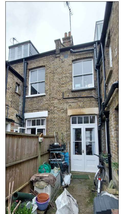
View of rear & side elevation (taken 2023)
