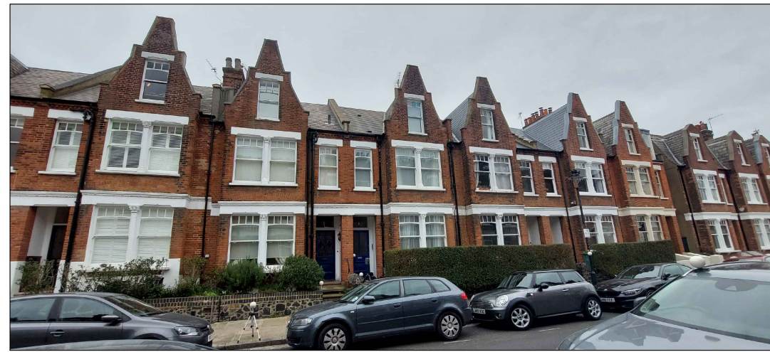
View of front elevation (taken 2023)
