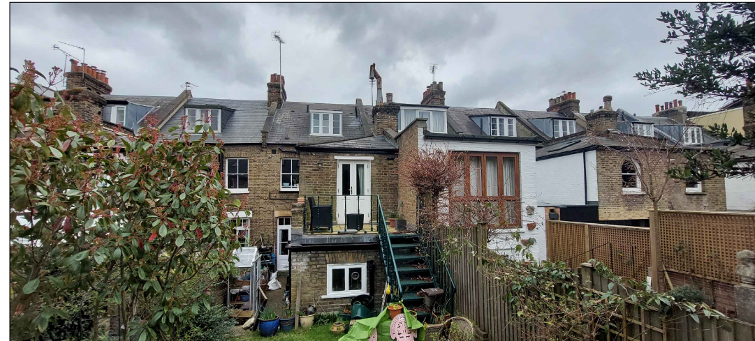
View of rear elevation (taken 2023)
