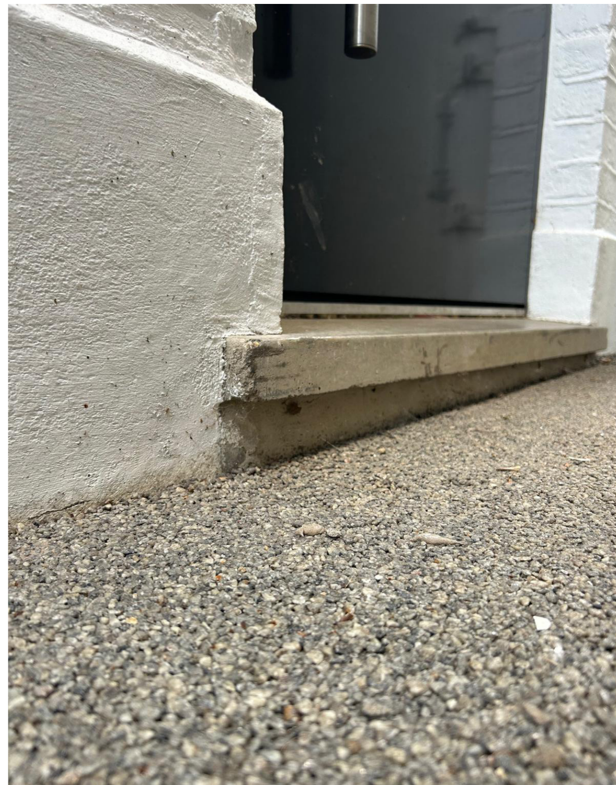
Front Door Threshold
