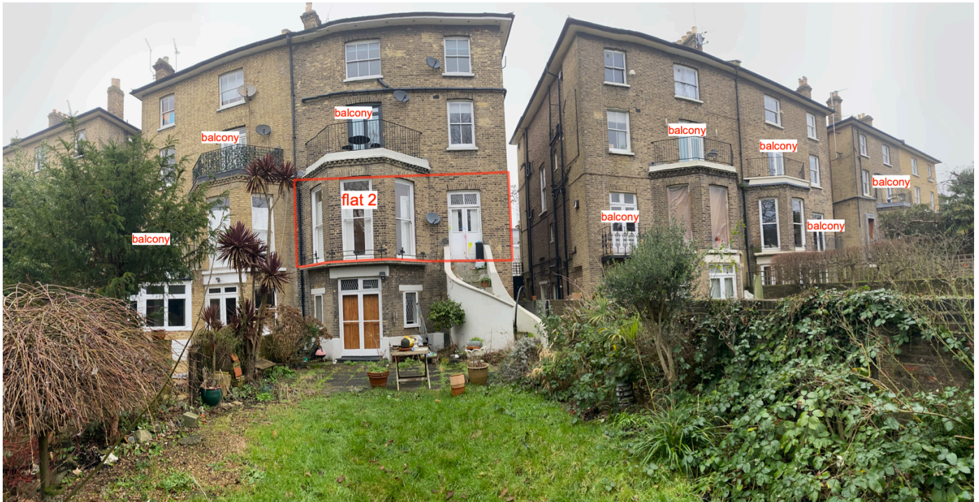
Rear View of No.99
