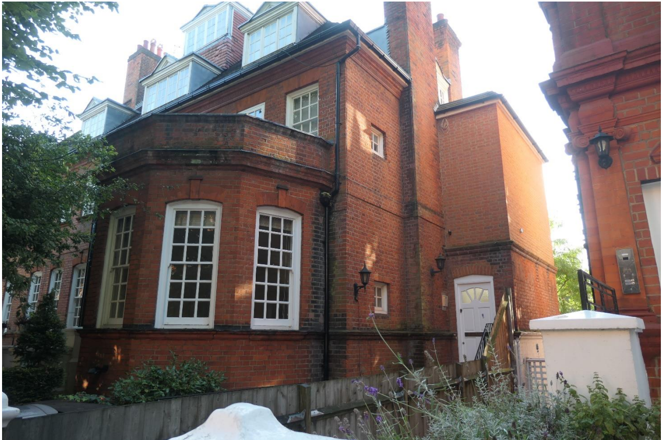
Photo 1: An oblique view of front and side elevation of 9 Wedderburn Road, showing the heightened side projection and the two tiers of dormers.
