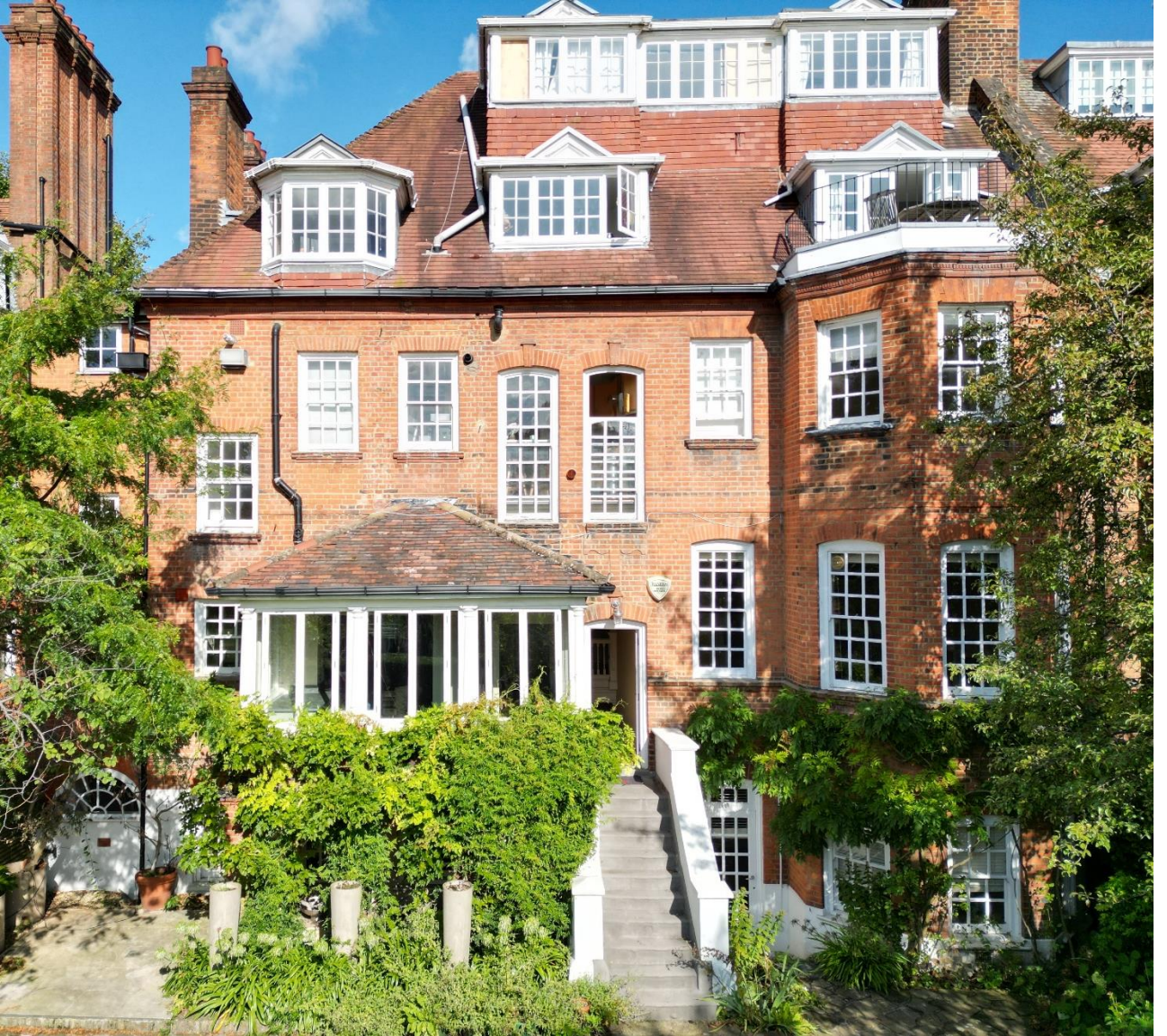
Photo 2: An elevated view of the rear elevation of 9 Wedderburn Road.
