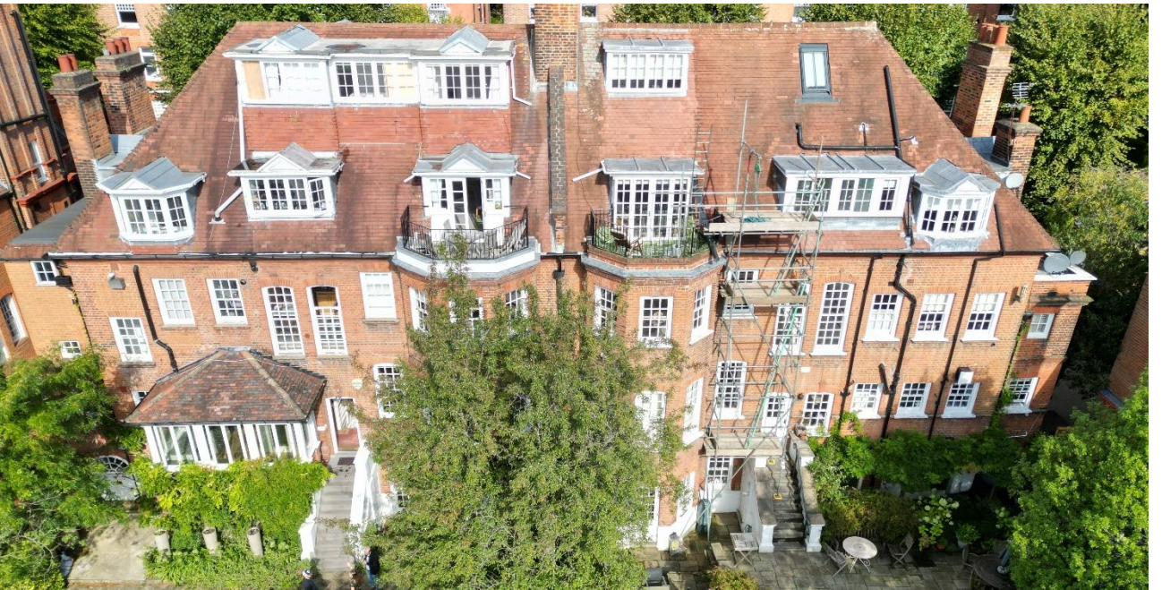
Photo 3: An elevated view of the rear elevation of 7 & 9 Wedderburn Road.
