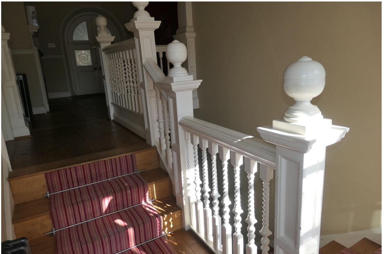
Photo 4: The main staircase is original (though not the treads and risers).
