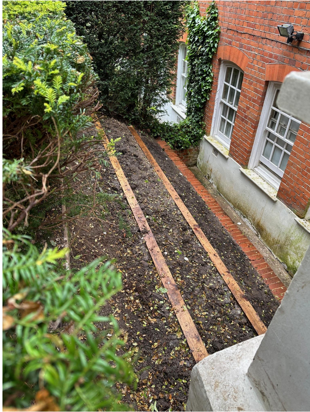
Lightwell - All plants have been removed
