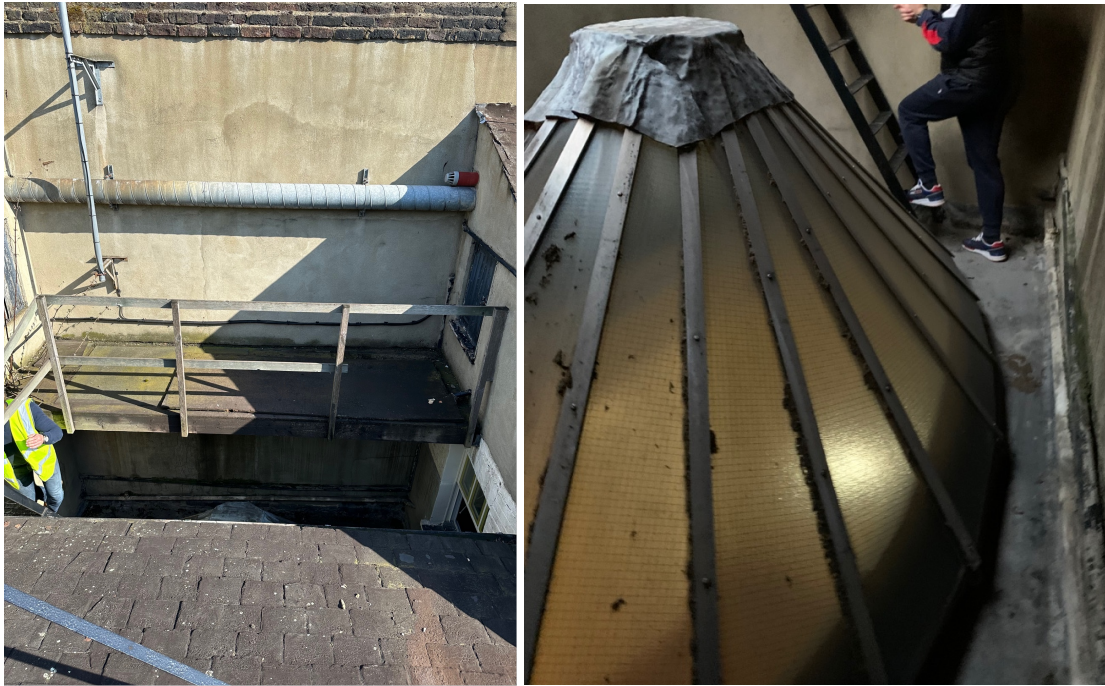
Photo of existing timber platform and skylights to be refurbished
