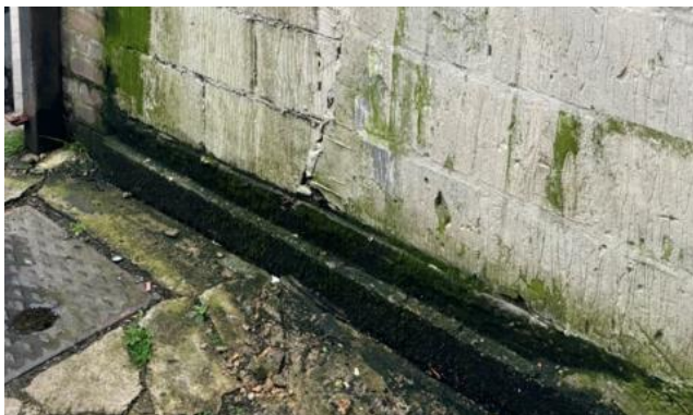
Figure 9: Ground floor concrete slab visible on the exterior of the building.
