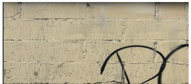
Figure 8: Concrete blockwork on East Elevation
