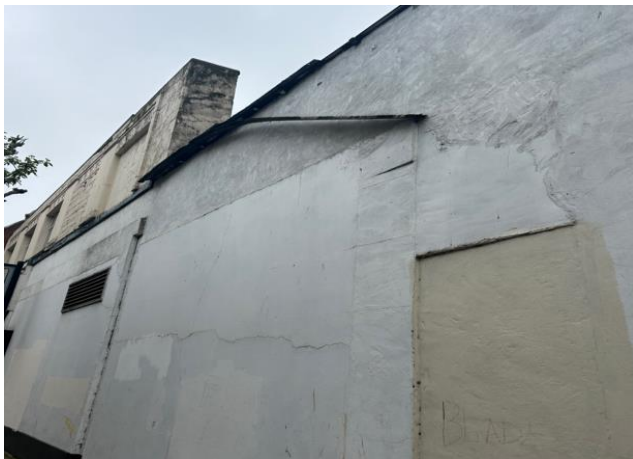
Figure 6: External brickwork covered in render on Southern Elevation
