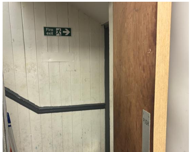
Figure 15: Timber door and timber clad walls
