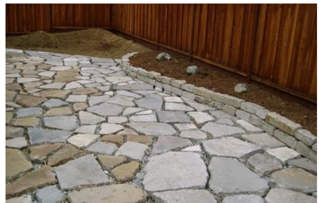
Figure 2: Reusing broken up concrete within landscaping, paving and kerbs is a good way to promote direct reuse onsite – Image: https://www.terranovalandscaping.com/90/
