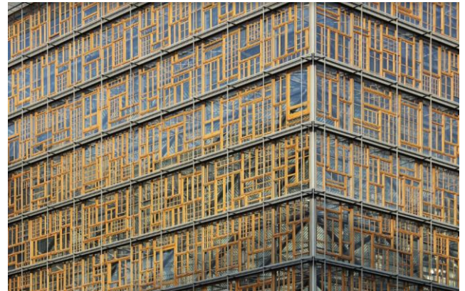
Fig 18 – EU Headquarters famously incorporates a patchwork of 3,750 recycled wooden window frames procured from
