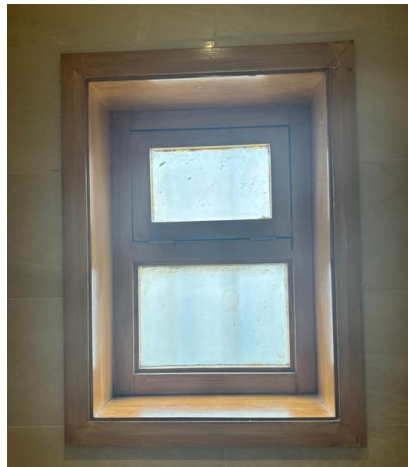
Timber framed windows in WC
