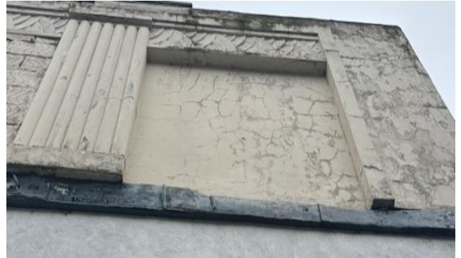
Figure 14: Stone Masonry on South Elevation
