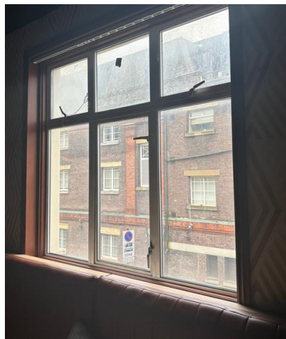
First Floor metal windows
