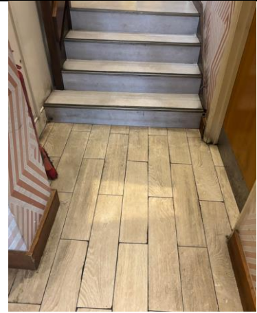
Stairs and hallway showing linoleum flooring
