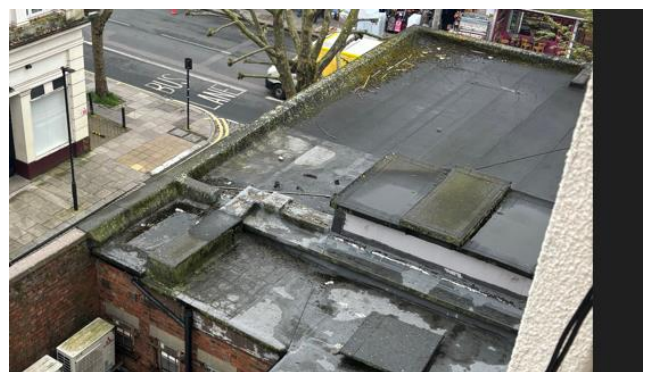
Figure 10: Bitumen Roof
