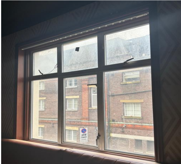
Figure 12: First floor metal framed windows
