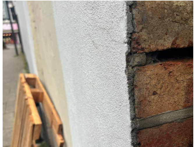
Figure 7: Close up on Exterior wall
