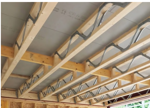
Picture of ceiling with exposed 'Posi-joists'.
