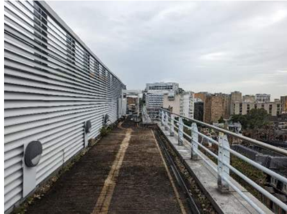
Photograph 2: Roof of 151 Shaftesbury Avenue, facing northeast.
